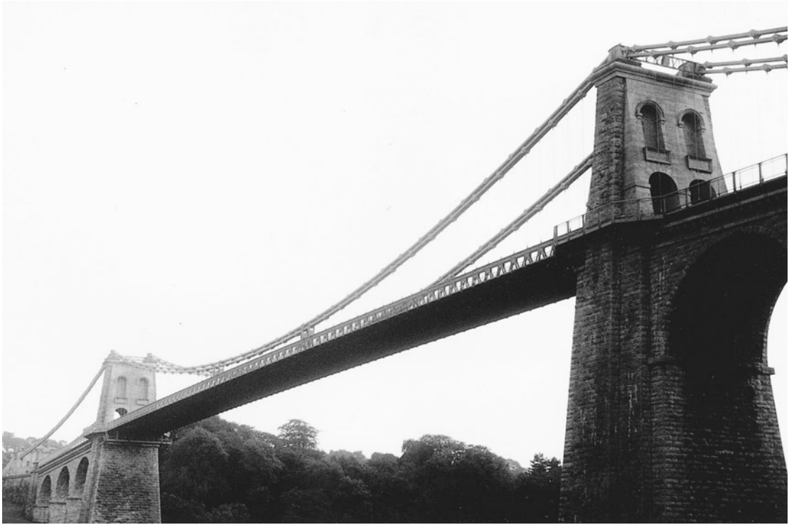
Fig. 14.4. Thomas Telford's iron bridge across the Menai Straits (completed 1824). In the eighteenth century, iron was adapted to structural engineering. The cast-iron arch bridge was followed by wrought-iron suspension bridges and wrought-iron tubular bridges. Organizational and managerial skills proved no less important for the success of bridge building than the technical mastery of iron as a construction material.
