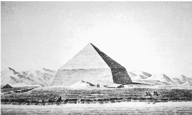
Fig. 3.4. The Bent pyramid. The lower portion of this pyramid rises at the same angle as the pyramid at Meidum, but ancient Egyptian engineers reduced the slope for the upper portion to ensure its stability. The Bent and Meidum pyramids were apparently constructed concurrently with engineers decreasing the angle of the Bent pyramid once they learned of the failure at Meidum.
