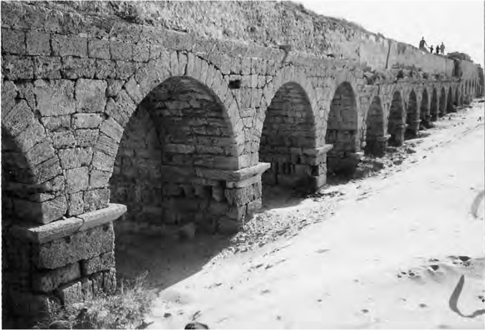
Romans constructed this aqueduct in 22 B.C.E. near Caesarea, a town now located in Israel between Tel Aviv and Haifa (photo by Paul A. Tucci).
