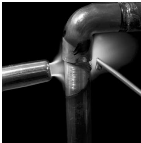
Solder is a metal alloy that is melted and then used for joining metals together. It is very useful in everything from plumbing to circuit boards.
