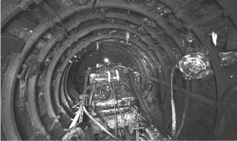
A compressor in a pillar mine tunnel.
