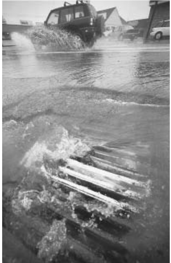
Storm drains overwhelmed by water following a heavy rain storm. AP/Wide World Photos. Reproduced by permission.
