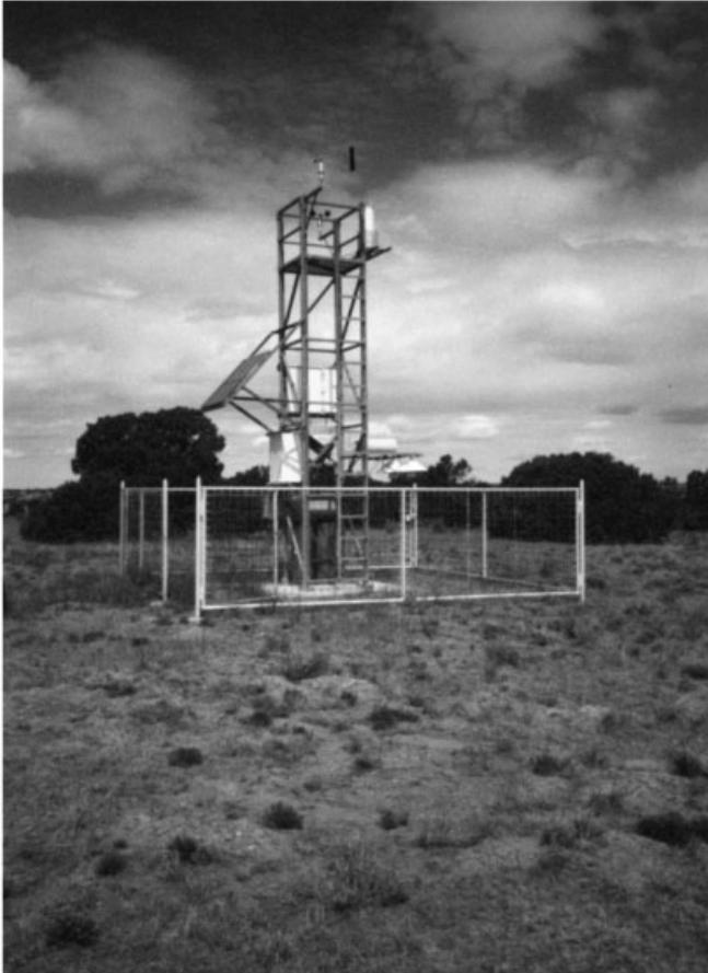
**Figure 21** Early remote automated meteorological observing system (RAMOS), late 1960s. See ftp site for color image.
