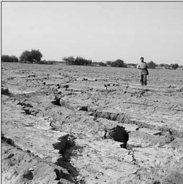
These cracks in the ground surface north of Chobari, India were caused by liquefaction induced during the Bhuj earthquake. (Image Copyright © James Mori, Research Center for Earthquake Prediction, Disaster Prevention Institute, Kyoto University)
