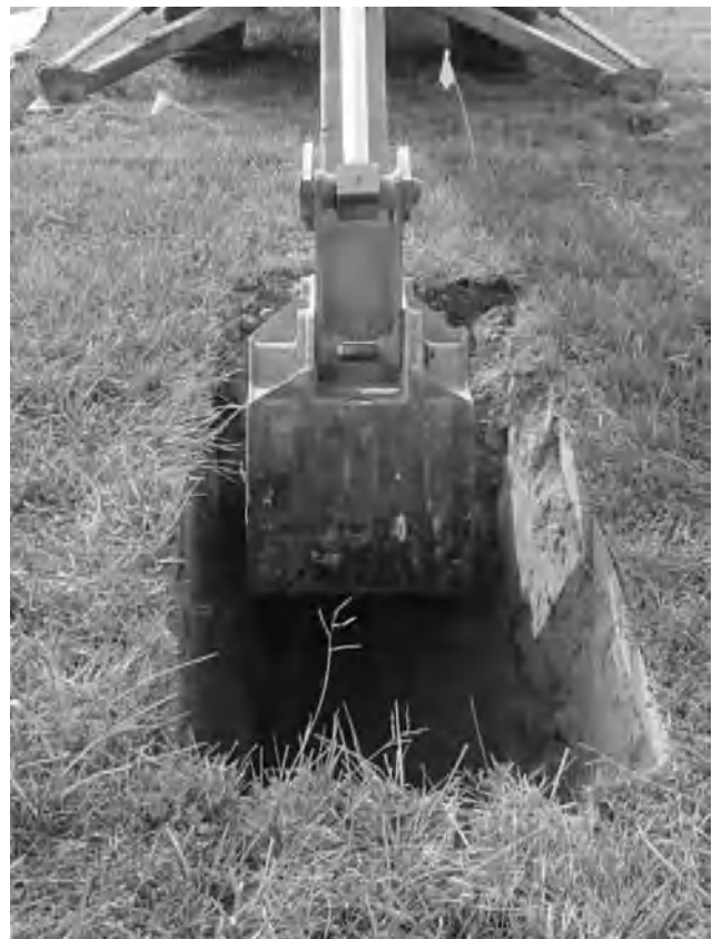
Figure 2. Backhoe digging trench for lysimeter installation.
