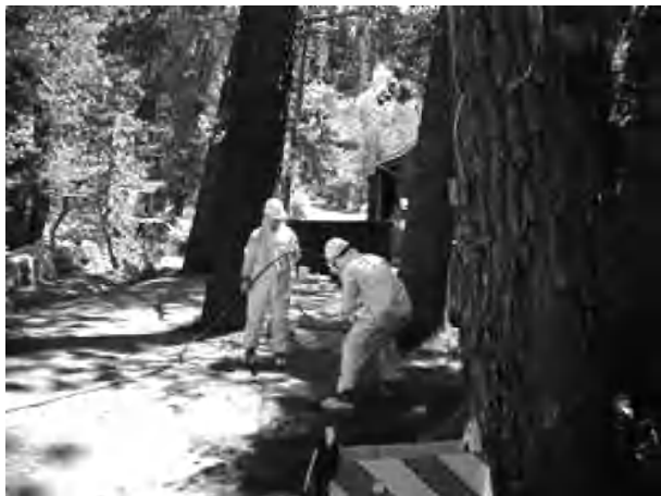
Figure 1. Handheld lances used to perform remediation by jetting technology in a limited-access site (FAST-TEK).
