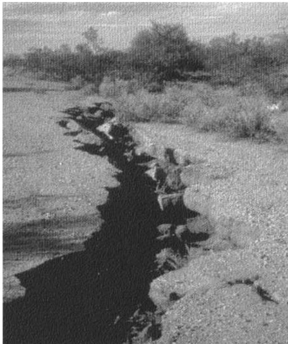
Figure 2. Pima County, Arizona. Sign warning motorists of subsidence hazard was erected after an earth fissure damaged a road in Pima County, Arizona (left photograph). Earth fissure near Picacho, Arizona (right photograph) (photographs by S.R. Anderson, U.S. Geological Survey).
