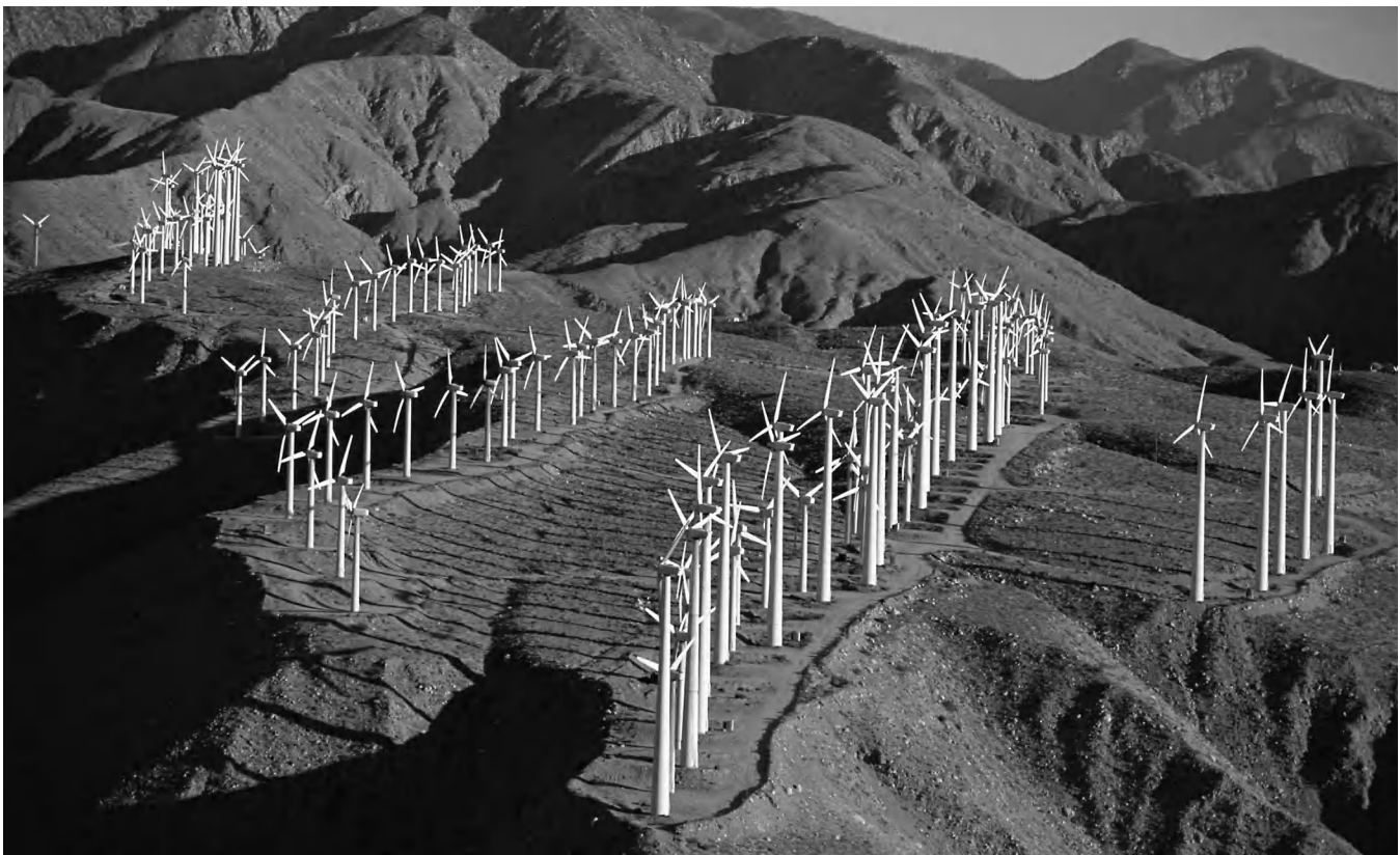
Projects like this wind farm in California may help the U.S. Department of Energy's Wind Powering America Initiative reach its goal of generating 5 percent of the nation's electricity through wind power by the year 2020.
