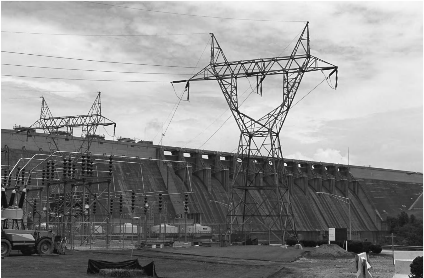
A hydroelectric plant in Tennessee. Once the water level reaches a high enough level, a gate is opened in the dam, allowing gravity to carry water down toward the generator. The force of the water falling spins the turbine and generator, creating electricity.
