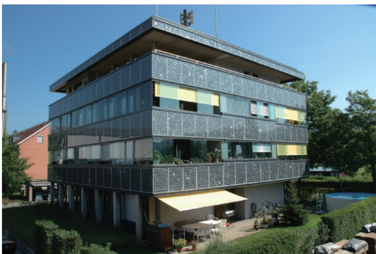
Figure 5.13 Photovoltaic facade system. Photo: SunTechnics.
