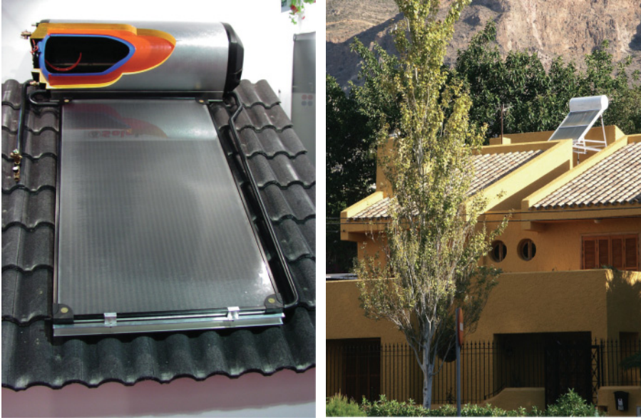
Figure 6.9 Left: Demonstration model of a gravity system. Right: Gravity system in Spain.
