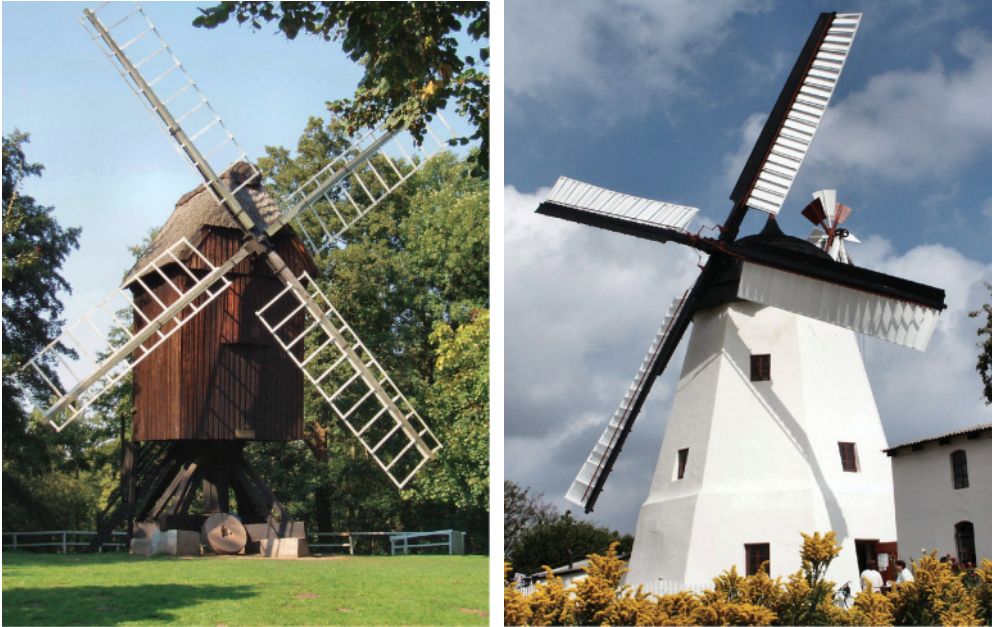
Figure 8.1 Left: Historical post windmill in Stade, Germany. Photo: STADE Tourismus-GmbH. Right: Dutch windmill on the Danish island of Bornholm.
