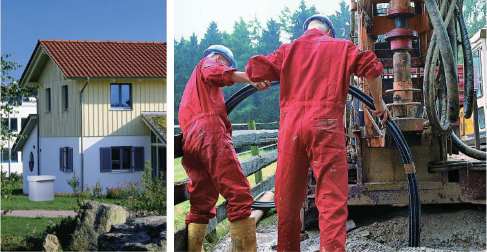
Figure 11.6 Air/water source heat pump installed outdoors and not requiring drilling (left). Deep drilling for a water/water source heat pump (right). Photos: STIEBEL ELTRON.
