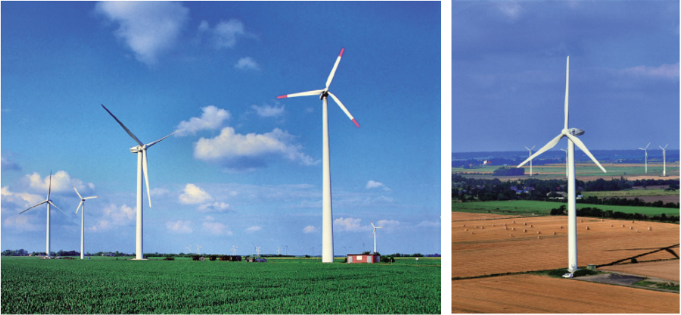
Figure 8.13 Wind parks. Source: REpower Systems AG, Photos: Jan Oelker.
