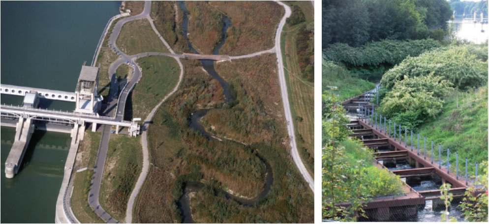
Figure 9.16 Left: Stream in the area of the Donaukraftwerk Freudenau power plant in Austria. Source: www.verbund.at . Fish bypass at Weserkraftwerk Bremen in Germany. © Weserkraftwerk Bremen GmbH.
