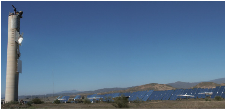
Figure 7.9 Research site for a solar tower power plant at Plataforma Solar de Almería (Spain).
