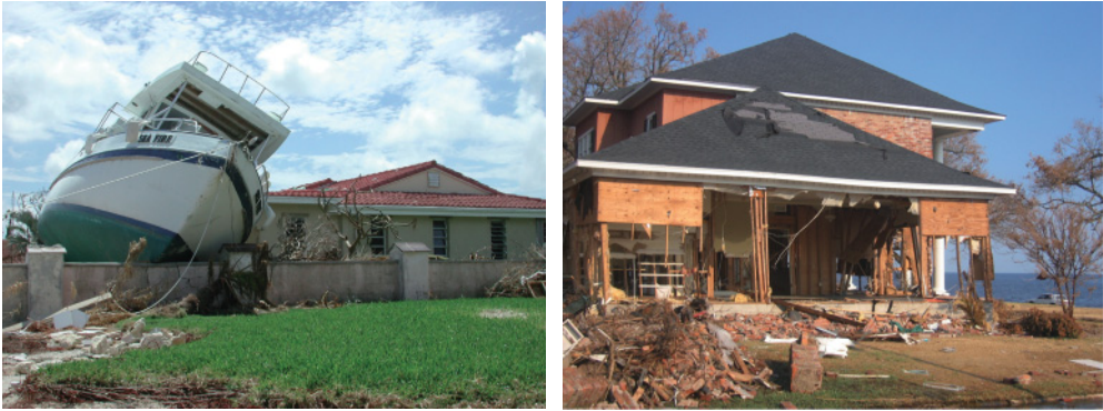
Figure 2.4 Damage caused by hurricanes in the USA. Photos: Munich RE Group.
