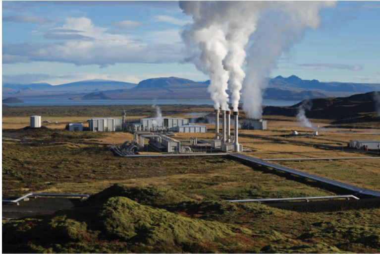
Figure 10.10 The Nesjavellir geothermal power plant in Iceland. Photo: Gretar Ivarsson.
