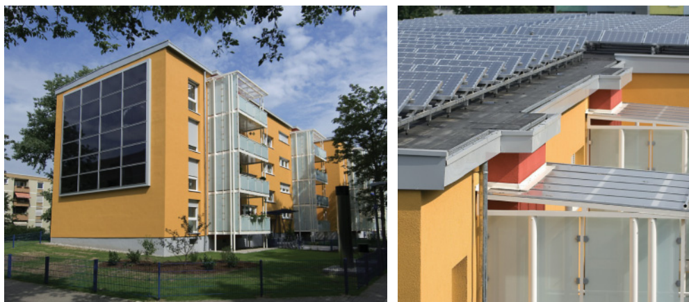
Figure 14.5 Constant hikes in energy bills are a thing of the past for this zero-heating cost house in Ludwigshafen, Germany. Source: LUWOGÉ, www.luwoqe.de .
