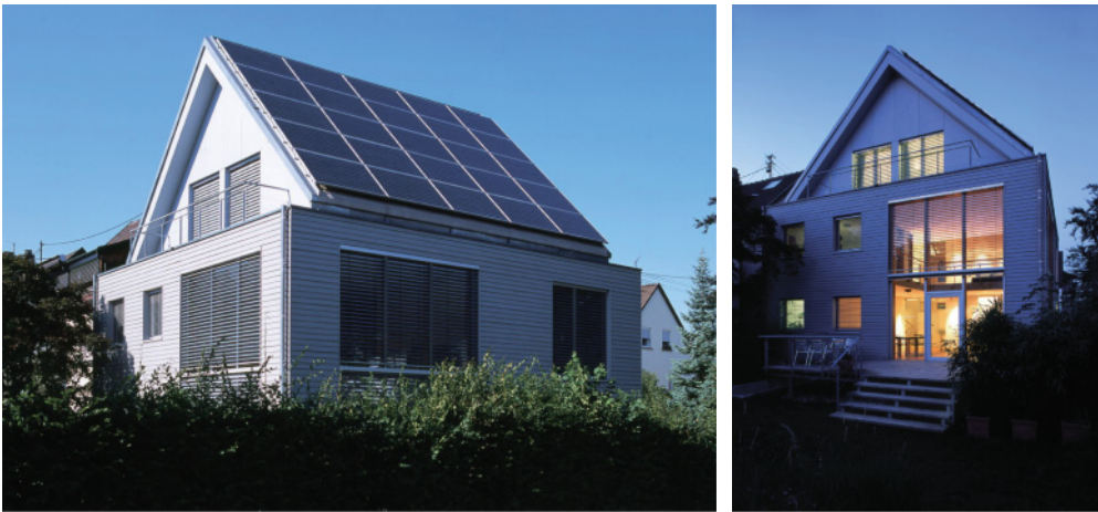
Figure 14.2 Plus-energy solar house in Fellbach. The photovoltaic system feeds more energy into the public grid each year than the house needs for its own heating and electricity. Source: Reinhard Malz, www.fellbach-solar.de .
