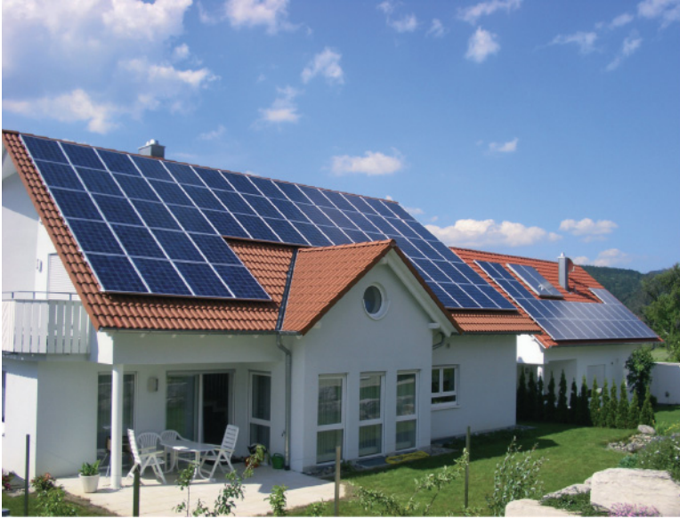
Figure 5.14 Photovoltaic systems on single-family homes. Foto: SunTechnics.
