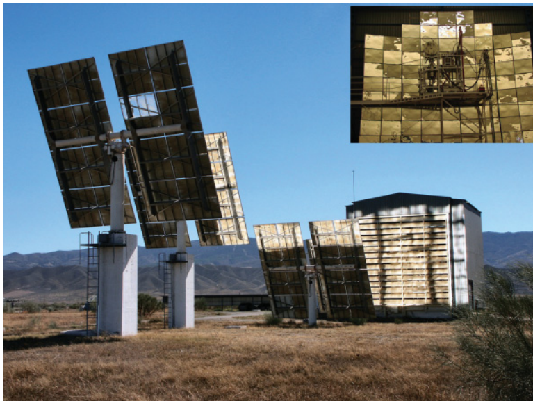
Figure 7.1 Solar furnace near Almería in Spain. Large tracking mirrors direct the sunlight towards a convex mirror (top right) in the interior of a building.
