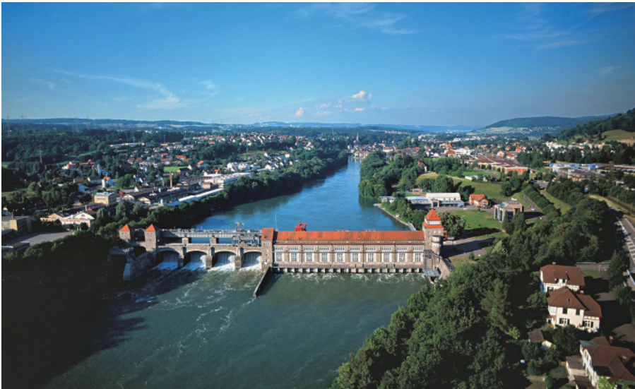
Figure 9.9 Run-of-river power plant in Laufenburg, Germany. Photo: Energiedienst AG.
