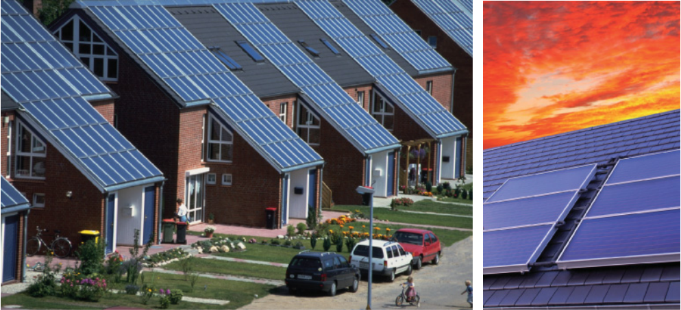
Figure 6.1 Modern solar thermal collector systems are an important alternative to conventional oil and natural gas heating. Photos: www.wagner-solar.com .
