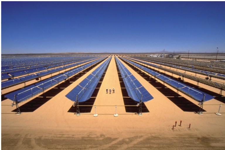
Figure 7.4 View of the Kramer Junction parabolic trough power plant in California (USA). Photo: Gregory Kolb, SANDIA.
