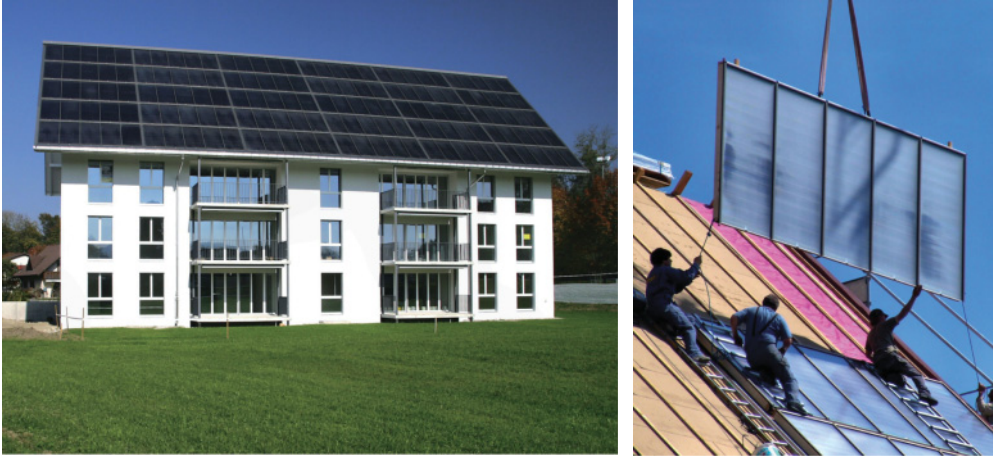
Figure 14.4 Left: First multiple-family dwelling in Europe to be heated 100% with solar thermal heat. Right: Installation of 276 m 2 roof-integrated solar collector. Source: Jenni Energietechnik AG, www.jenni.ch .
