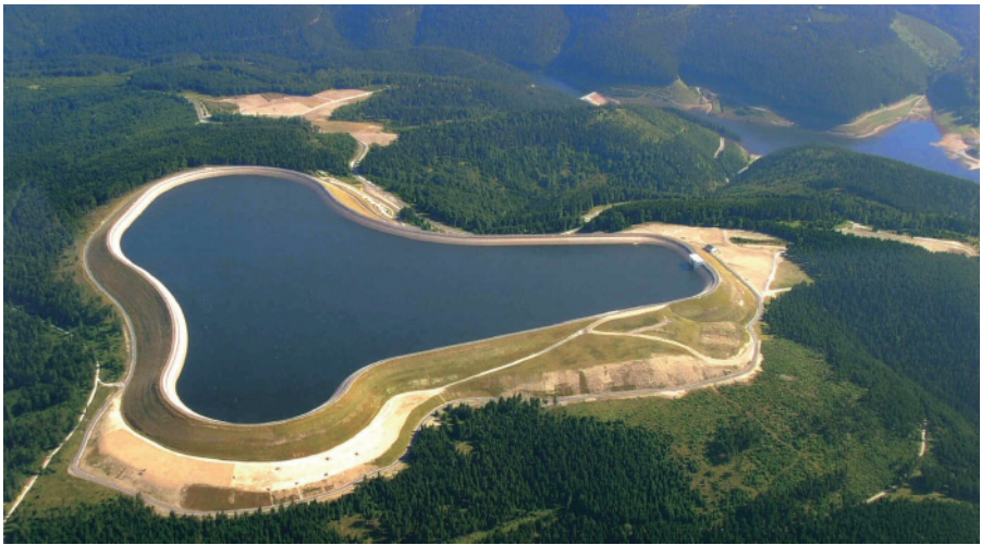
Figure 9.12 The Goldisthal pumped-storage power plant in Germany. Source: Vattenfall Europe.
