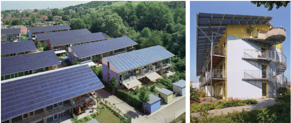
Figure 14.3 Schlierberg solar housing estate in Freiburg, Germany, with 50 plus-energy houses. Source: Architekturbüro Rolf Disch, www.solarsiedlung.de .
