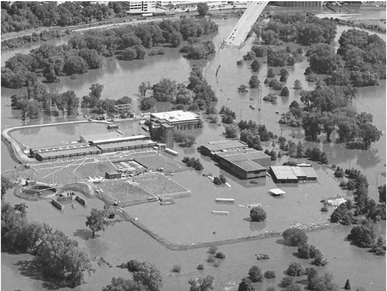
This water treatment plant in Des Moines, Iowa, was flooded by the Raccoon River in 1993. Flooding was a serious problem all over the United States that year due to rainfall amounts far above average. AP/Wide World. Reproduced by permission.
