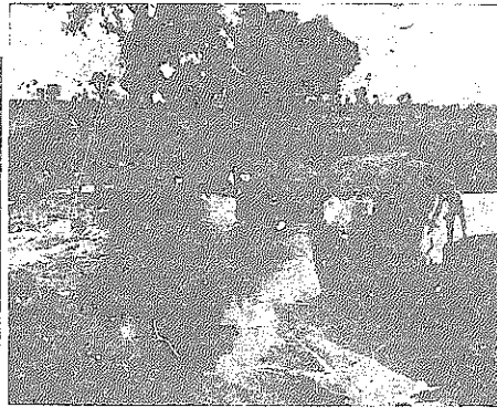
In the absence of adequate cross-drainage works on roads, loaded bullock-carts have to experience much difficulty in crossing streams that flow over the roads.
