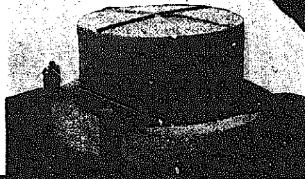
Fig. 2. Single unit biogas plant designed by Shri J.J. Patel of Poona Agricultural College.
