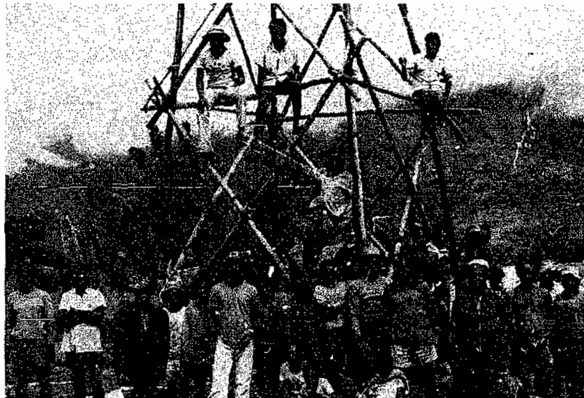
Fig. 2: Local Construction Crew
