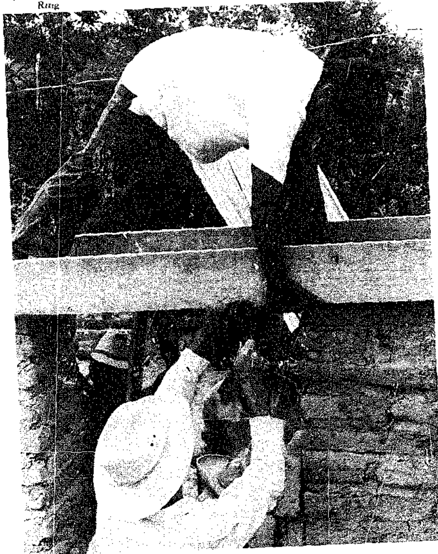
Fig. 5. A Construction Team Making the Wooden Form for the Concrete Reinforcing Ring
