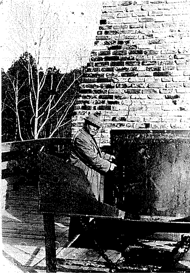
PLATE 20 Professor Ray Farabee indicates the charging point of the old Tannehill furnace. Professor Farabee was the furnace master for the refring of the old furnace.
