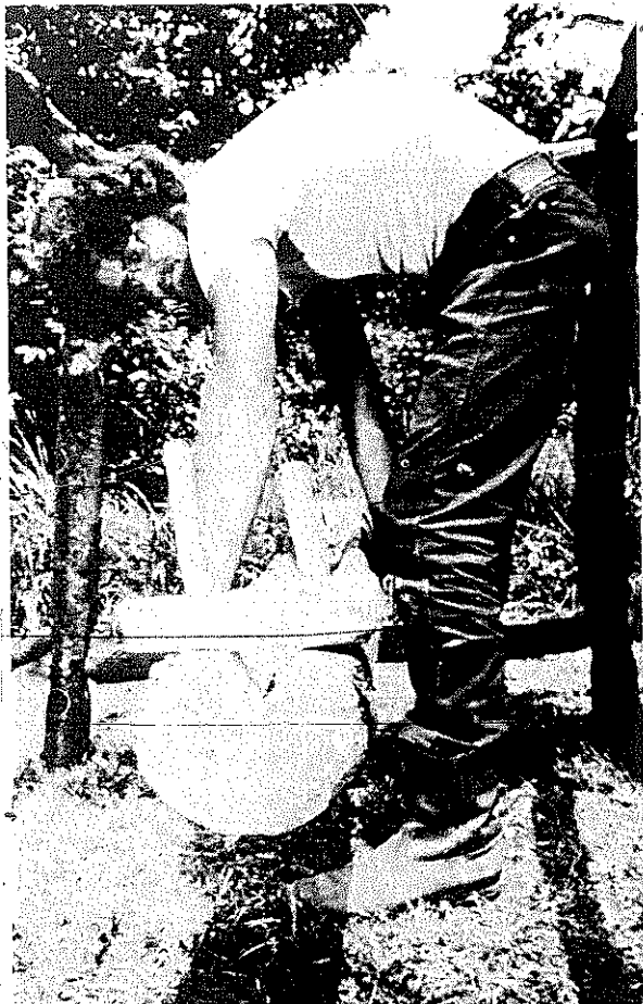
PLATE 205 Laying the drain trough. A foot adze and hatchet were used to hew the trough. (Photo by Pete Lindsley.)
