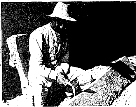
Figure 198 Mason Smoothing Stone with Kernel Hammer
