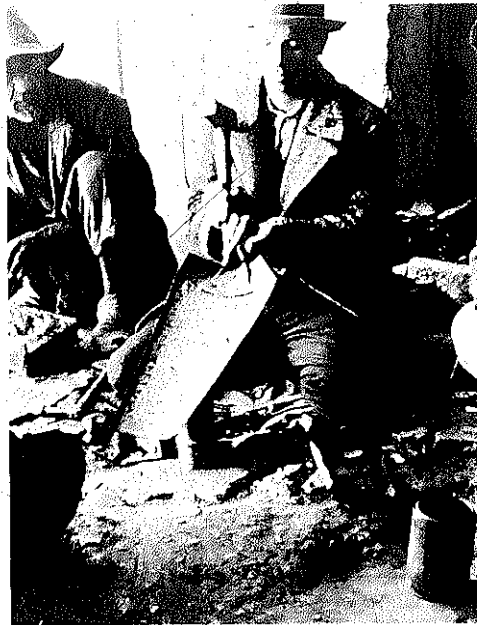
Figure 70 An Anvil Set in the Ground
