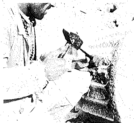
Figure 199 Mason Chiseling Flutes
