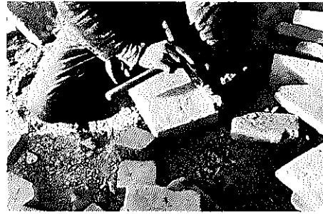
Figure 182 Marking Bricks for Edge Trimming
