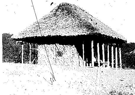
Figure 159 A Peasant House near Rūdbār Gilan
