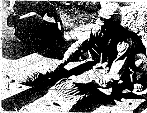
Figure 234 Beating Clay into the Mold
