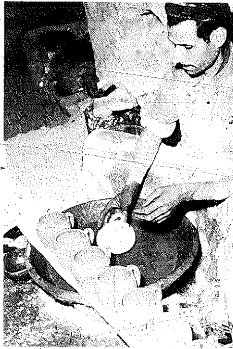
Figure 245 Applying Glaze by Dipping
