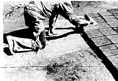
Figure 173 Emptying the Brick Mold
