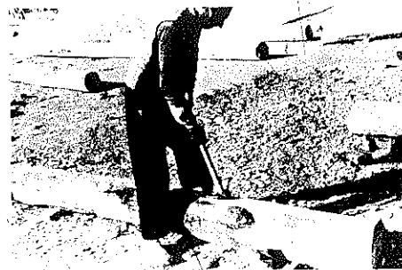
Figure 113 Trimming a Log
