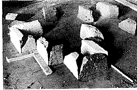
Figure 186 Cut Bricks Laid out on the Tracing Surface
