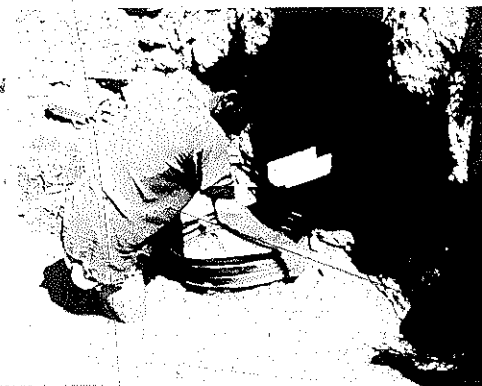
Figure 171 Straining the Slaked Clay
