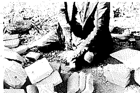
Figure 183 Trimming the Brick Faces
