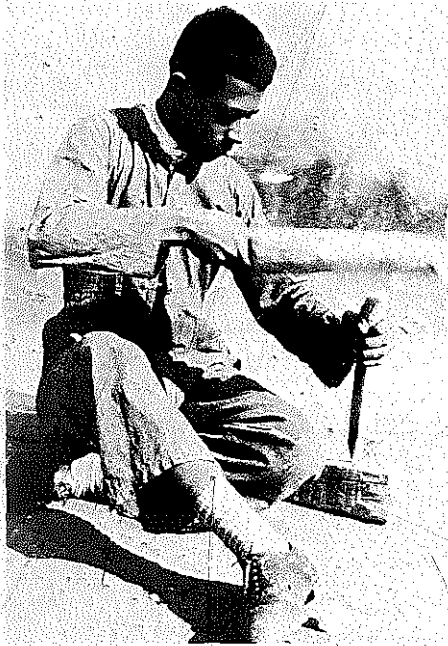
Figure 123 A Mortise Chisel and Mallet
