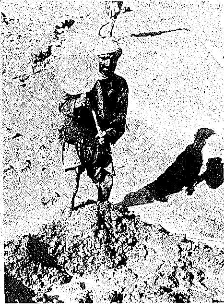
Figure 162 Preparing the Loam for Mud Bricks
