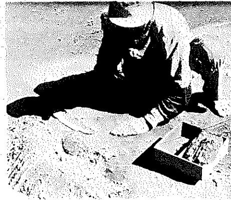
Figure 172 Filling the Brick Mold
