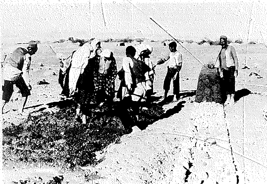
Figure 161 The Building of a Pisé Wall
