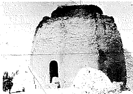
Figure 175 An Open Brick Kiln
