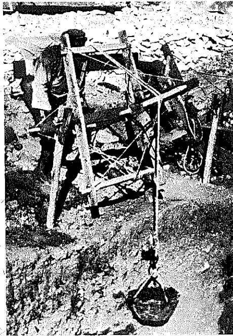
Figure 163 A Windlass above a Loam Pit
