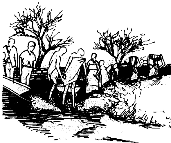
Construction work involving the whole village.
