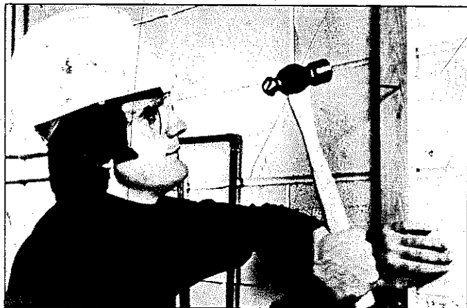
Use a heavy ball-peen hammer for driving special hardened nails into masonry. Note the hard hat and the safety goggles. Hand Tools Institute Photo.
