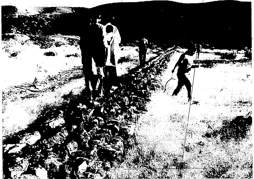
Sahel zone, NIGER: A stone dam for the purpose of retarding the floods in a wadi bed near the missionary station of Tschirozerine (near Agadcz). Such dams are being set up by paid teams of workers who are supposed to tend them later on. Often the force of the floods was underestimated and the dams broke. Now, a new program was started to dam up the water of small wadis in order to improve the natural vegetation and to utilize the flooded areas for agriculture.
