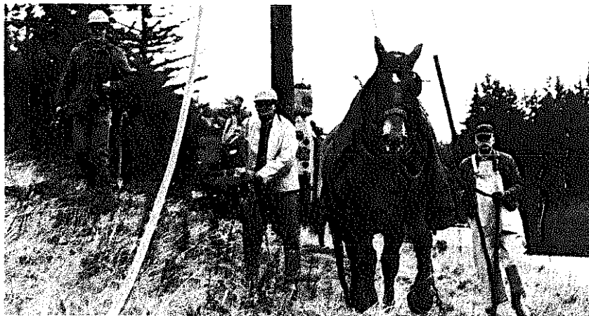
Fig. 1-4. Another example of one of the many specialized roles that the draft horse can fill is this draft horse being used to unroll telephone cable in the state of Washington.
