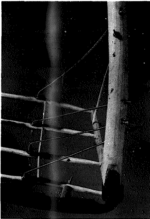
The supporting all-thread strut is bolted in place with a wing nut.
