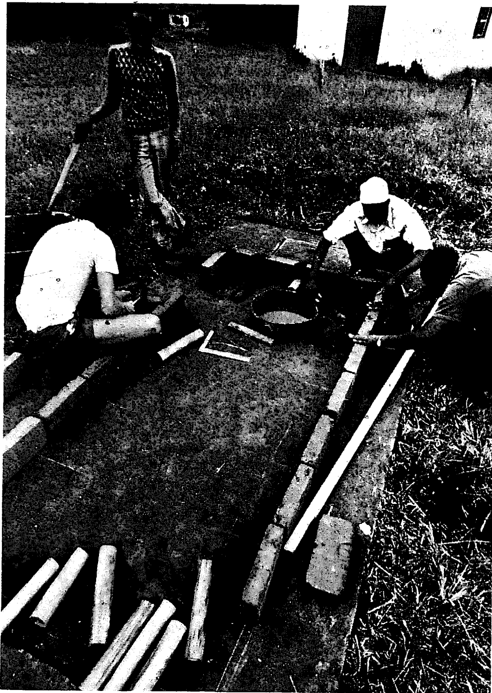
Early construction of Model 2 Solar Dryer
