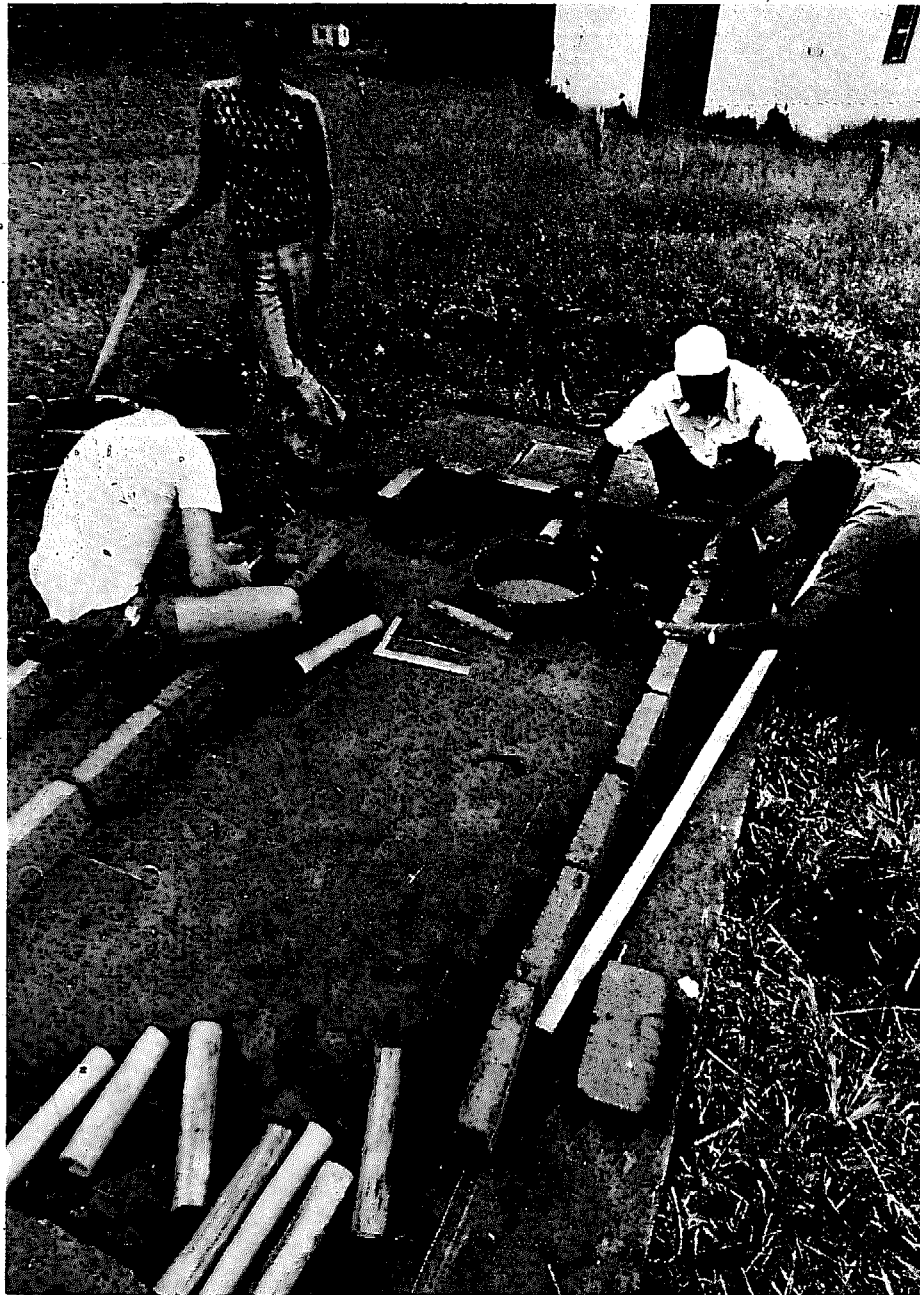
Early construction of Model 2 Solar Dryer
