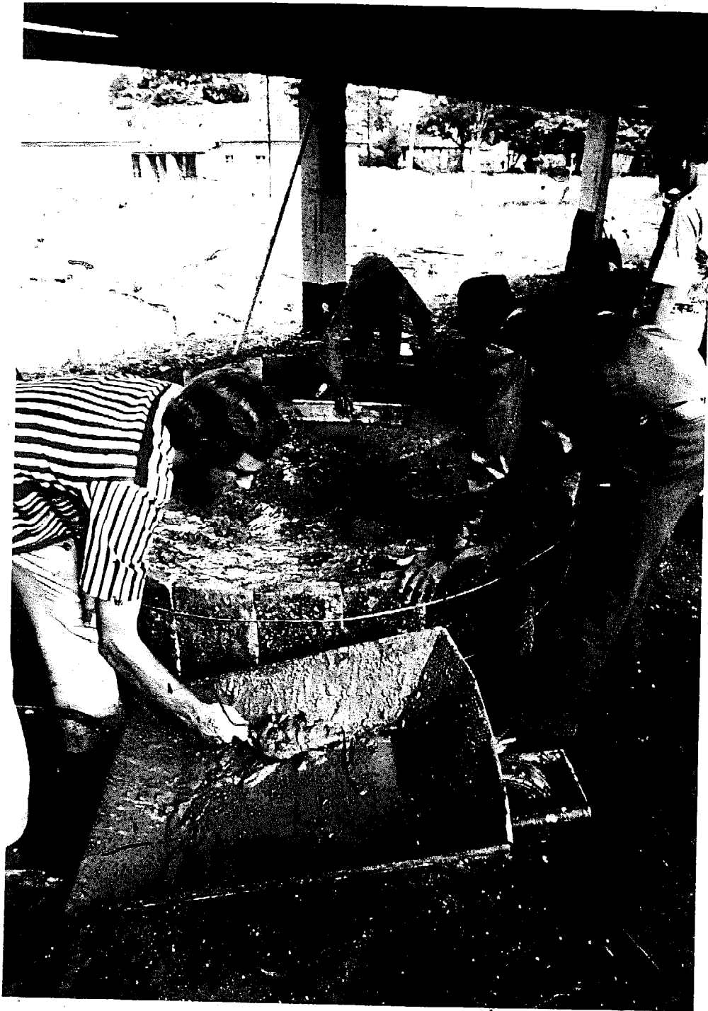
Photo – Erik Bentzen 4 cm of concrete poured and tamped before placing re-rod armature; then covered with another 6 cm layer of concrete.
