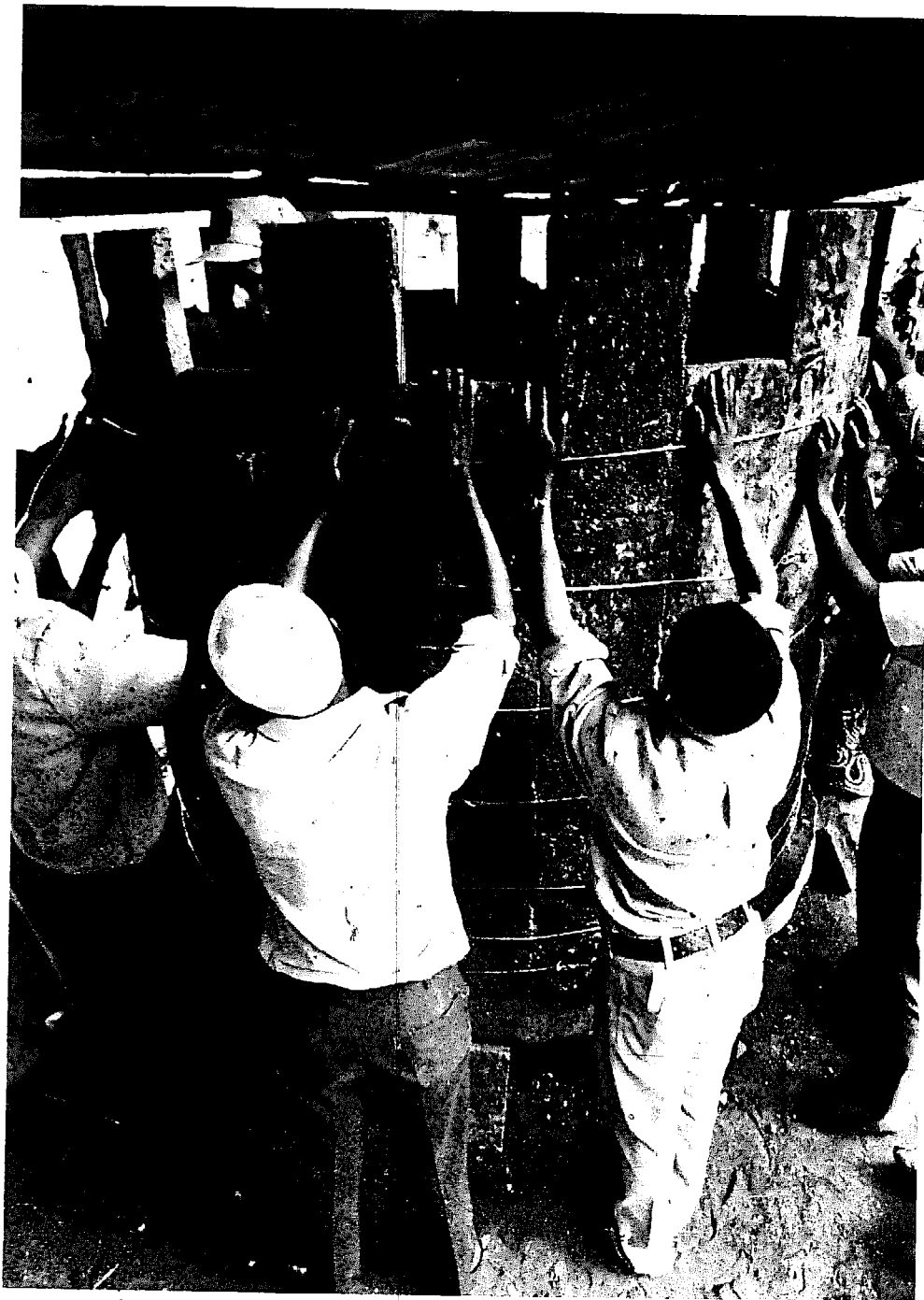
Photo – Erik Bentzen Mounting the wall: In addition to 91 large staves and 26 small ones, one roll of 3 mm galvanized wire (4 kg) and 10 wire tighteners are needed.
