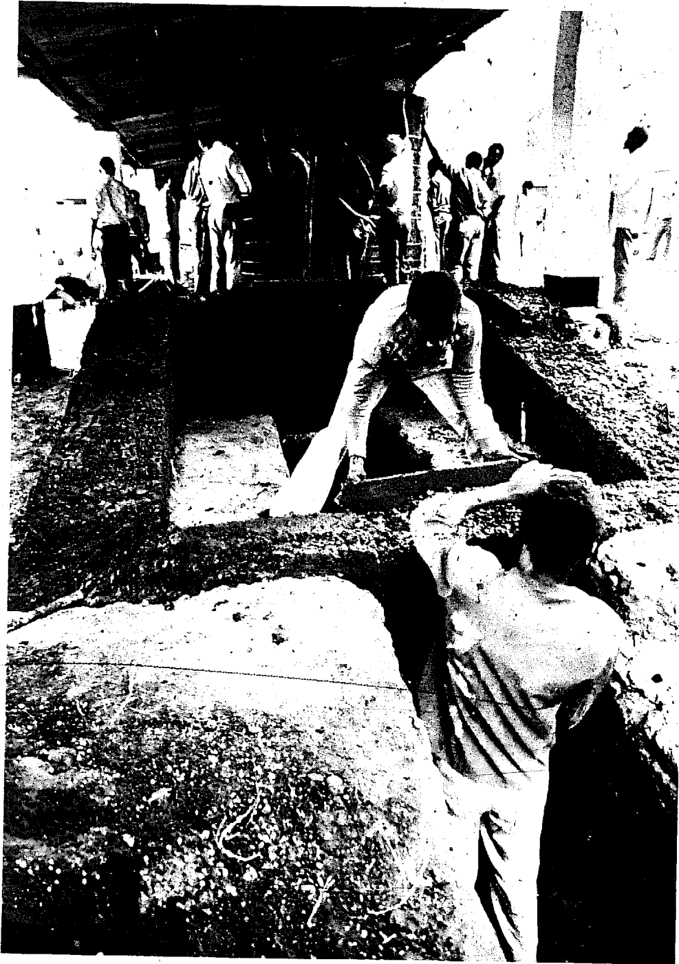
Photo – Erik Bentzen Mounting the dryer walls. (In the background is a nearly completed 4.5 ton cement stave silo.)
