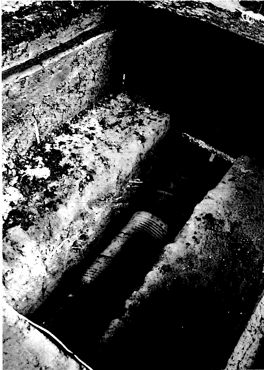
Placing the fire box barrels.
