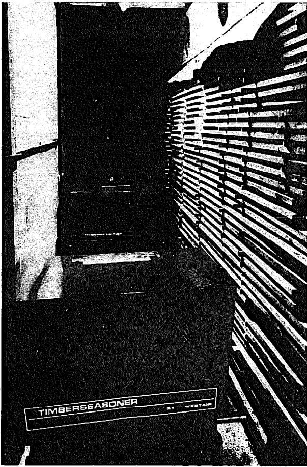
Plate 5 Dehumidifiers in a forced draught timber drier
