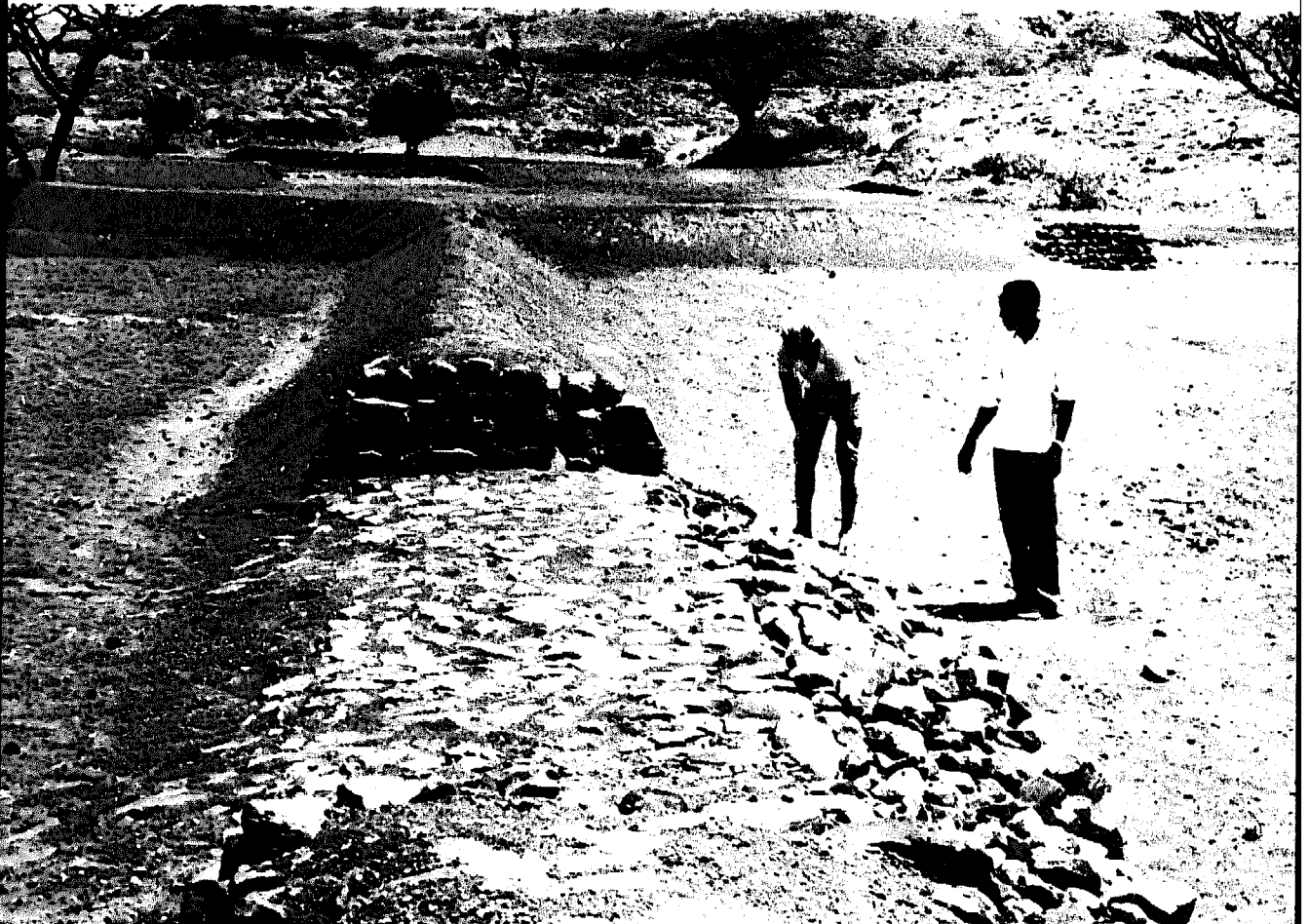
Plate 14. Detail of gabion spillway construction in a bund system — part of the River Naupwala water harvesting scheme, near Lokitaung, Kenya.
