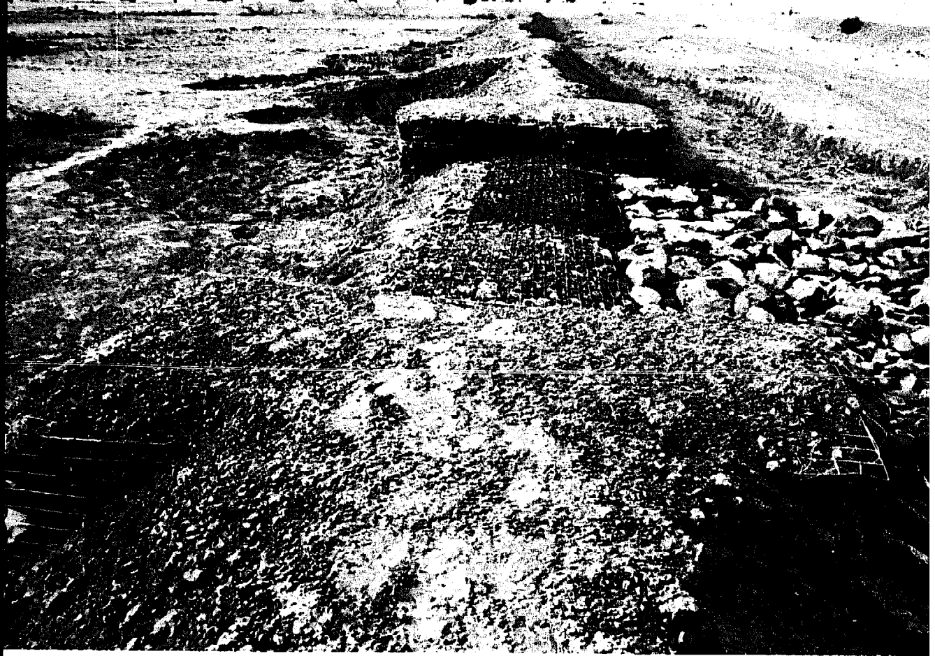
Plate 13. One of a series of water-harvesting bunds built with gabion-reinforced spillways, near Lokitaung, Kenya.
