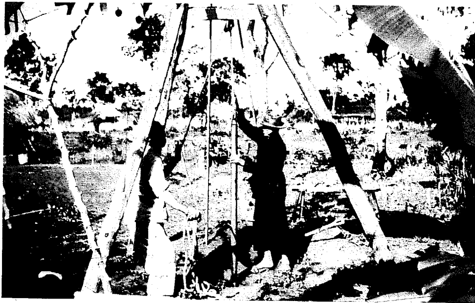
Fig. 19 Bailing well with 6 cm diameter bailer
