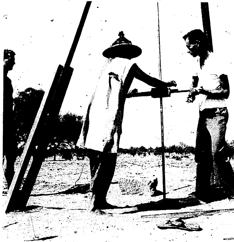
Fig. 11 Drilling with a helical auger
