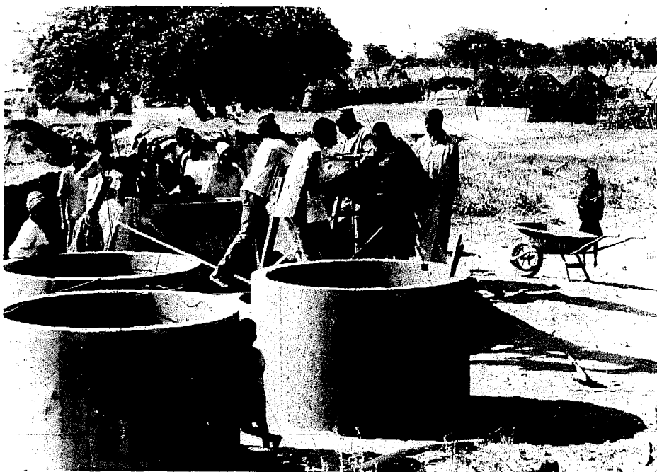
Fig. 51. Caisson sections made with commercially fabricated mould (Note perforations in surface to admit water)
