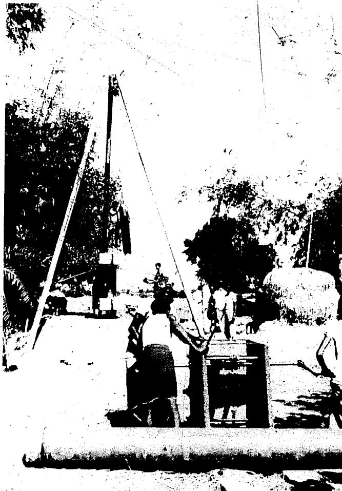
Bailing well with manpower
