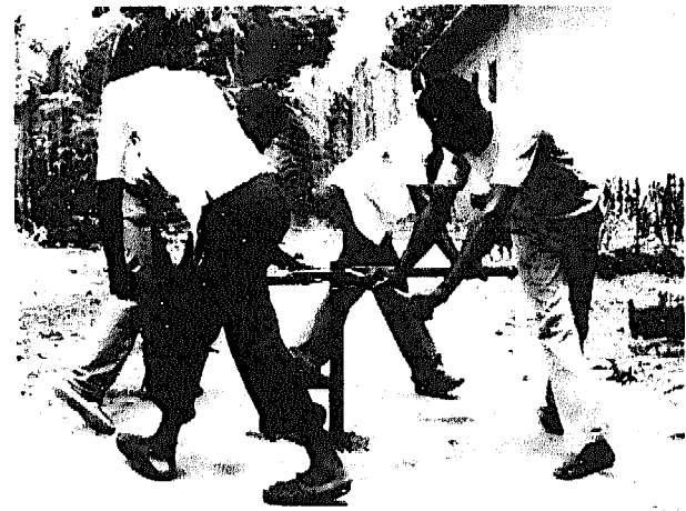
Fig. 45. If the soil is too hard, the heavy-weight set can be used.
