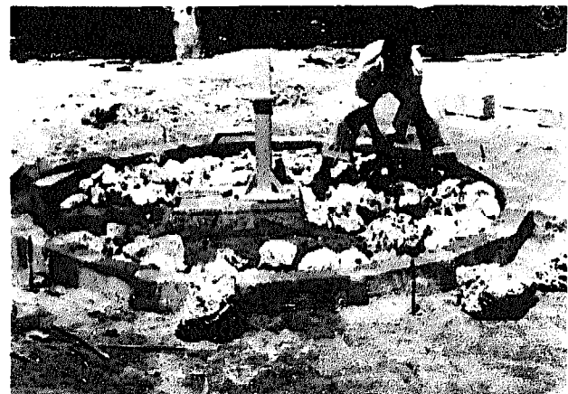
Fig. 111. Stones are broken down to the proper size. Note the opening in the rim for the spill water outlet.
