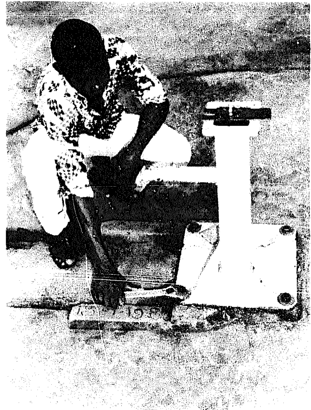
Fig. 131. The pump stand is fixed onto the concrete cover. The pumprod is prevented from falling by a catcher.
