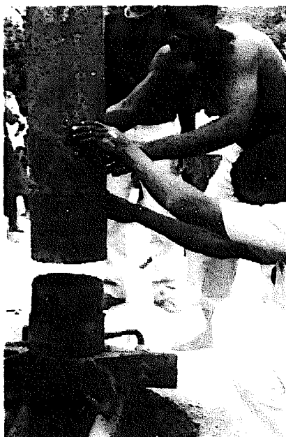
Fig. 69. A casing section ready to be screwed onto the previous one.
