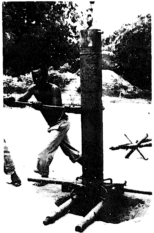
Fig. 89. Casing sections are unscrewed by means of a chain spanner.
