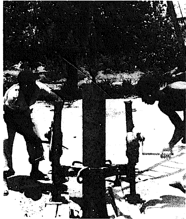
Fig. 91. Overloading of the tripod can be avoided by pulling up the casing with jacks.
