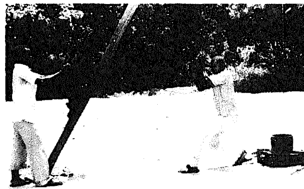
Fig. 71. Bailing in coarse sand or gravel. The winch operator should exactly follow the instructions of the person who is bailing.
