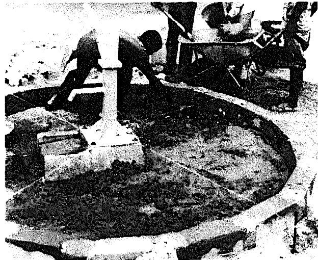
Fig. 110. Laying a foundation of mortar for the hardcore.
