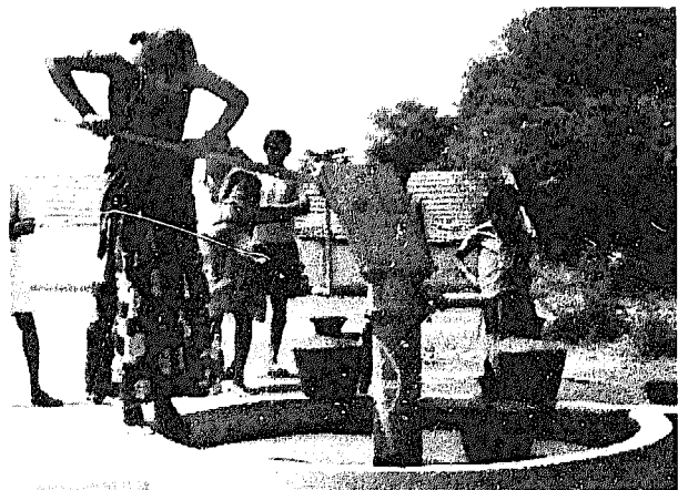
India Mark II handpumps presently serve more than 200 million people. The standard design requires both skill and effort when downhole components need maintenance. Modified designs aimed at simplifying maintenance are being tested in the Handpumps Project.
