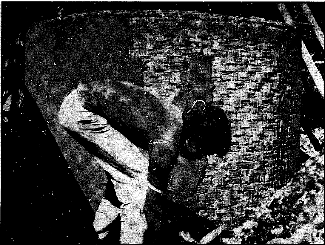
A nearly completed bamboo-cement tank: a technical success
