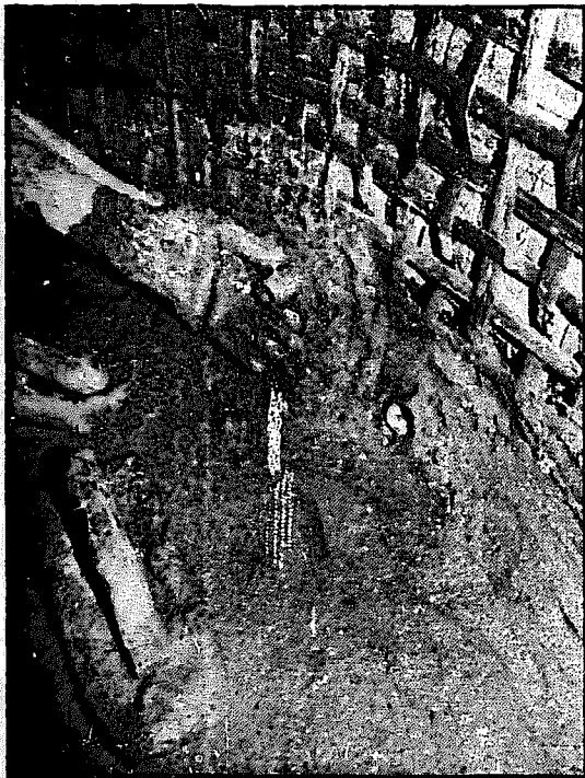
Left: internal plastering of the tank floor Right: applying plaster with rubber gloves
