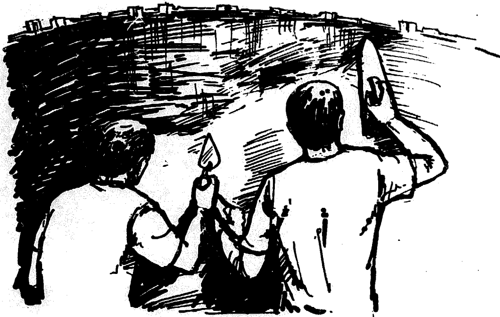
A second coat of plaster is applied with masonry trowels
