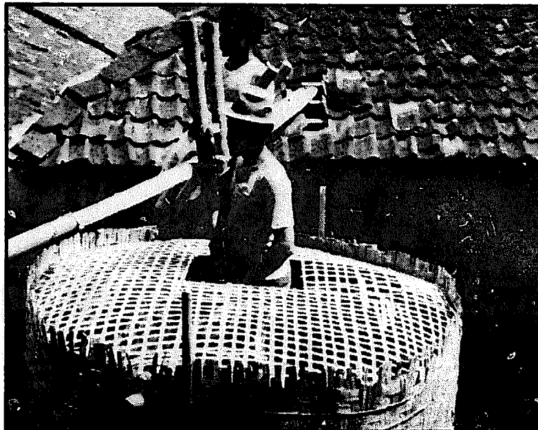
scaffolding for easy entry and exit
