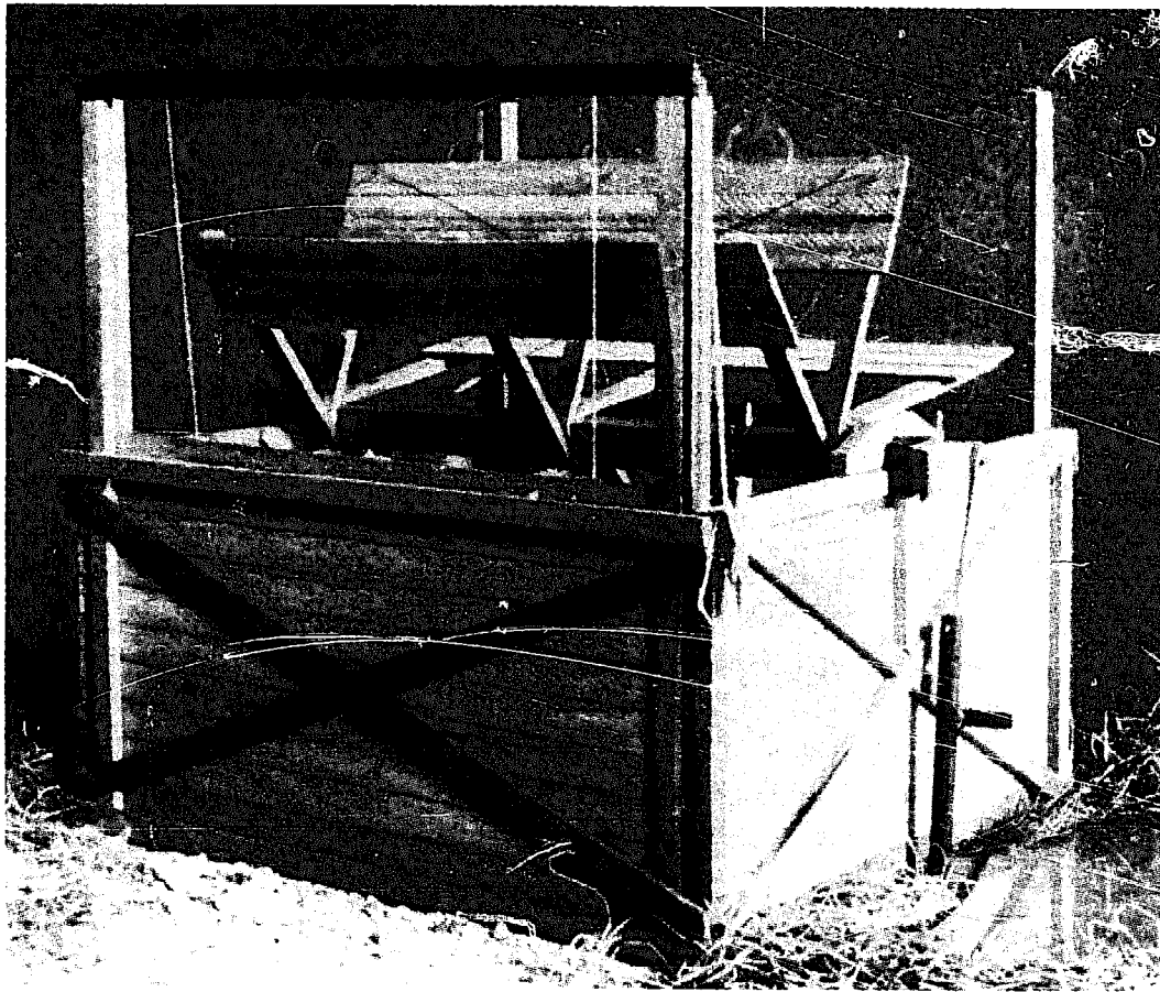
FIGURE 21 Model of a jumbo windmill with wind guard or cut-off. [Source: Barbour, Ref. 5]
