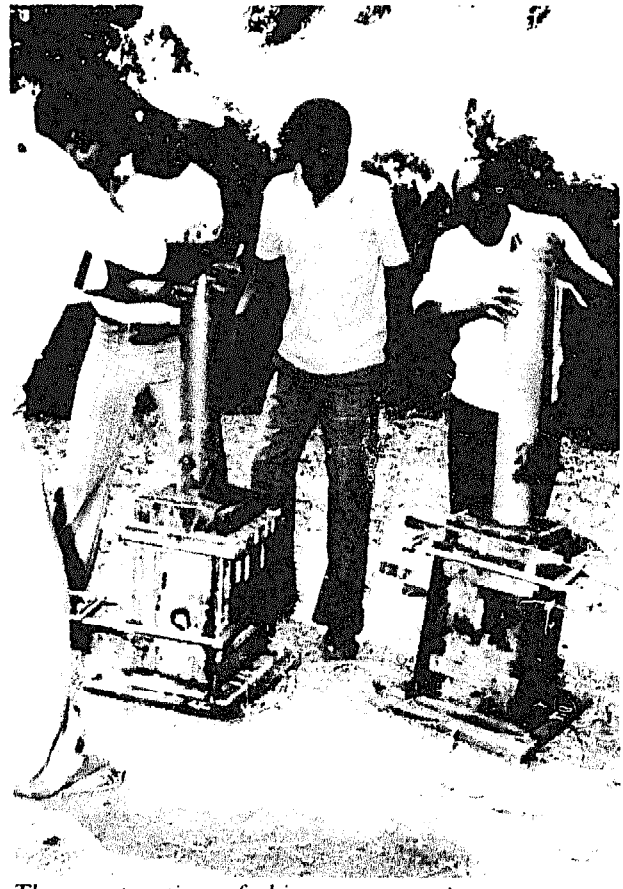
The construction of chimney segments.
