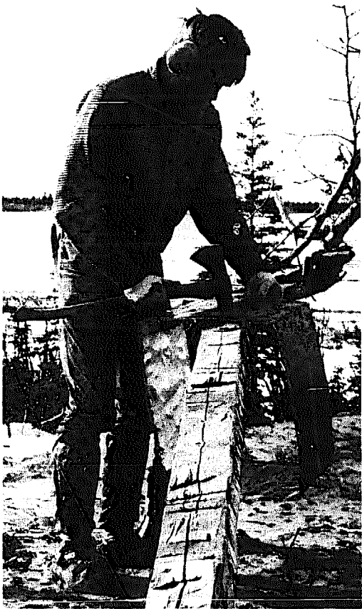
Figure 13.10—Forming the stove body on a squared log.
