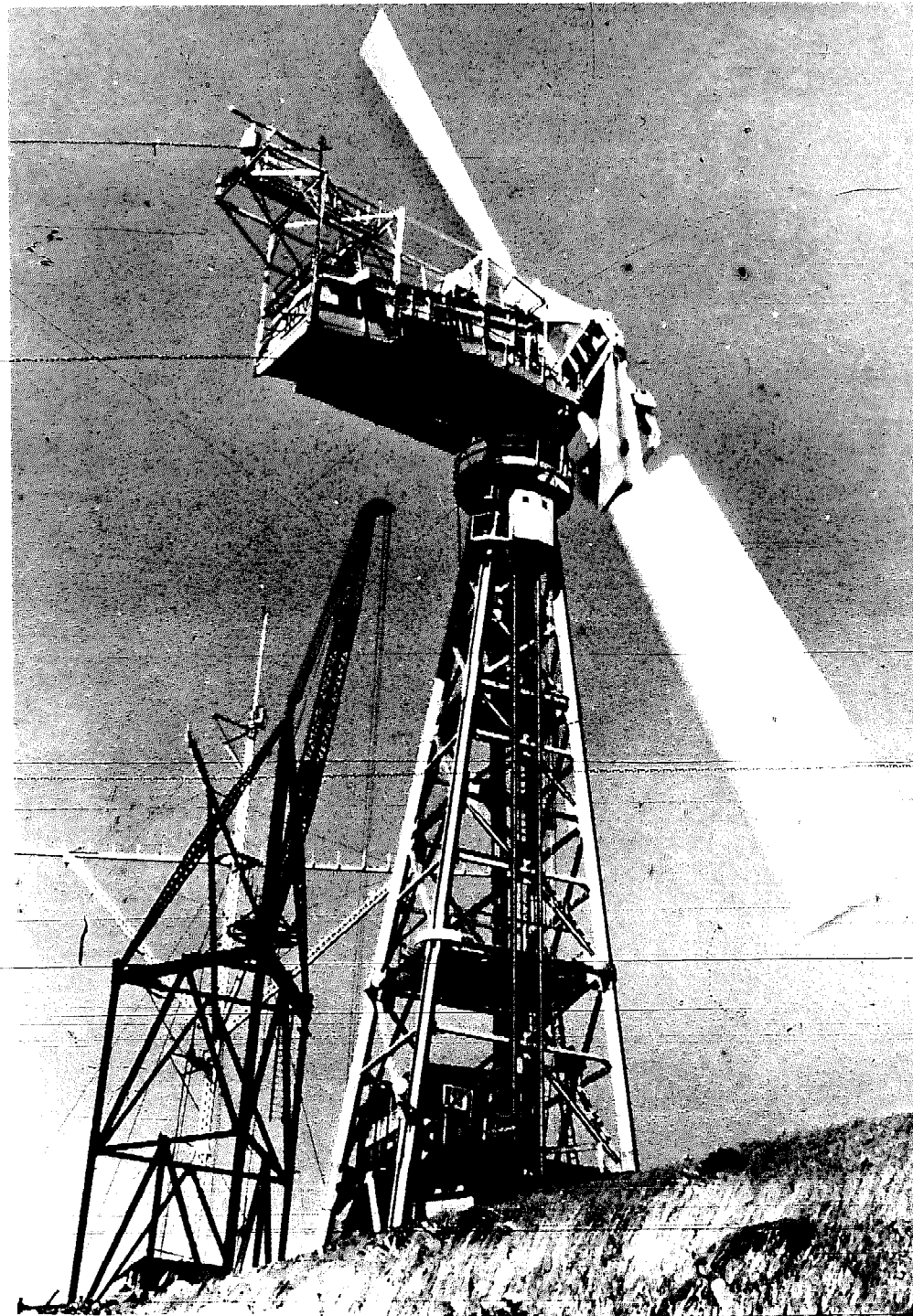
Rated at 1250 kilowatts, the giant Smith-Putnam Wind Generator produced electricity for the Vermont power grid during World War II.
