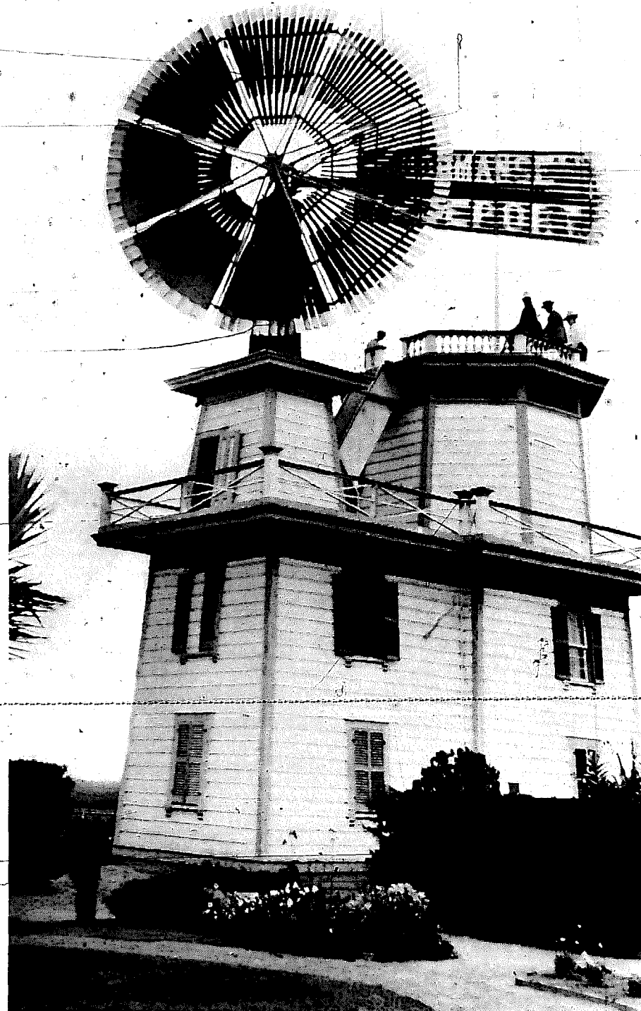
A water-pumping windmill of early California. The storage tank was built into the structure itself.
