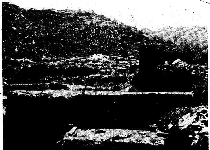
Fig. 18. The Bishband powerhouse.
