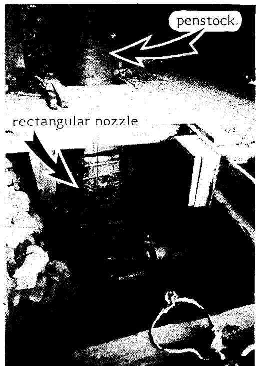
Fig. 16. A view of the turbo-generating area below floor level at the Lillonai (1) powerhouse. The last oil drum used in the penstock is tapered to form a rectangular nozzle leading to the turbine (under wooden cover). Also visible is the generator and separate exciter.
