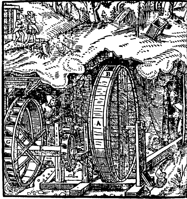
fig. 43: Ventilating air pump.
