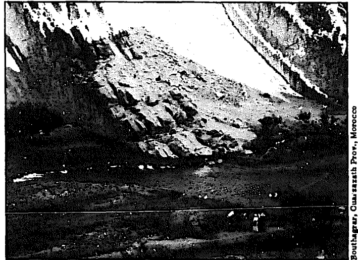
Fig. 5.44. Intake to a traditional irrigation canal. Despite the fact that the beginning of the canal is oriented nearly parallel to the stream, a rock outcropping deflects water toward the right bank during the river's high stage. The temporary weir would also wash away.
