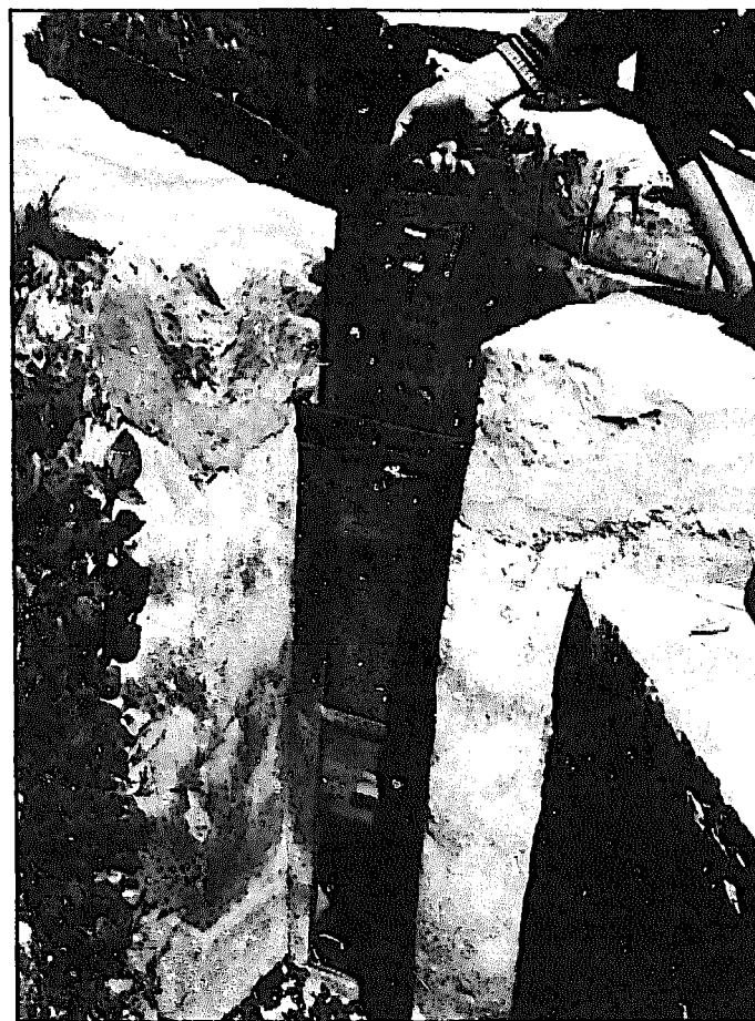
Fig. 5.173. A small sliding gate.
