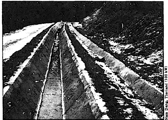
Fig. 5.83. A drainage ditch to the right of the power canal collects runoff and diverts it under the canal at several points along its length. The power canal here has not yet been put into operation.
