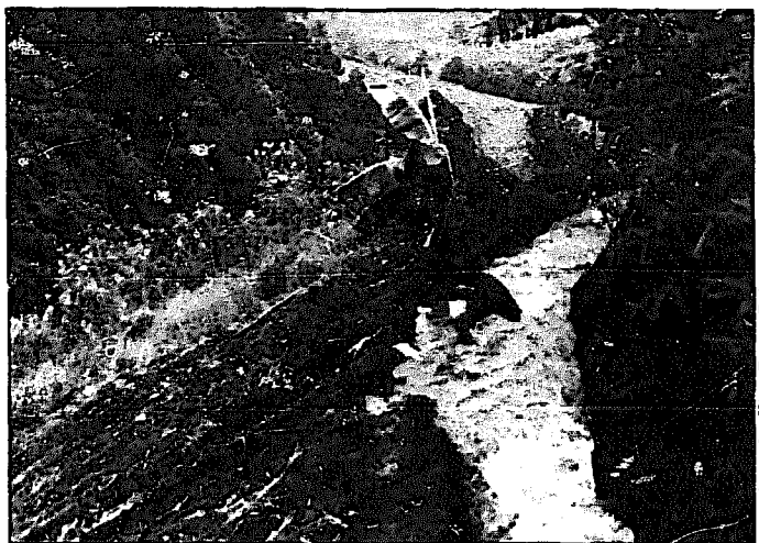
Fig. 5.85. A canal with inadequate freeboard can overflow and start eroding the downhill slope. This problem is frequently aggravated by people who use the banks of canals as footpaths.
