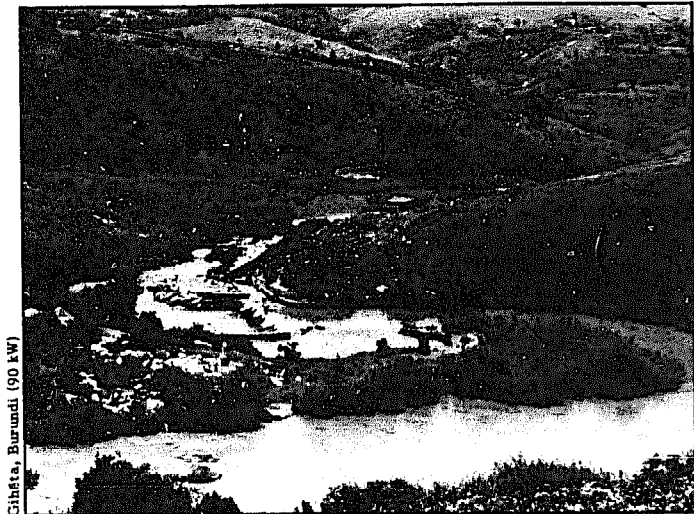
Fig. 5.34. After construction of the weir was started from the right bank, streamflow began eroding the left bank at the oxbow. As a result, a right angle bend in the weir was subsequently incorporated to reach the firmer rock foundation on the left bank slightly downstream (also see Fig. 4.24).
