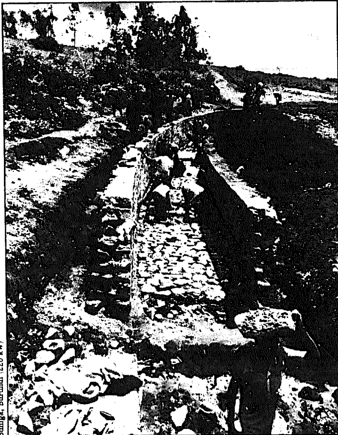
Fig. 4.22. With the canal walls largely completed, stone masonry is being laid for the base of the canal. Before the wall and canal bottom in the foreground can be completed, a small drainage ditch will be placed underneath.
