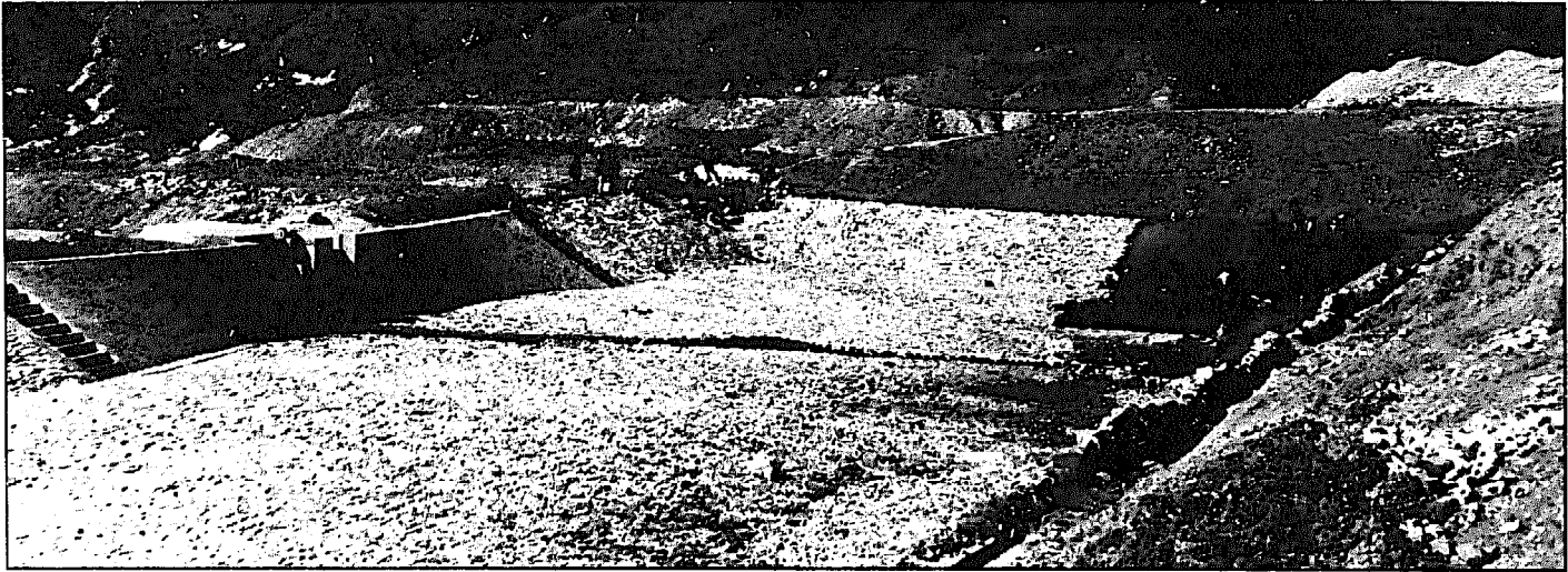
Fig. 5.122. Close-up of the forebay under construction. Concrete is used only in the vicinity of the inlet to the penstock.
