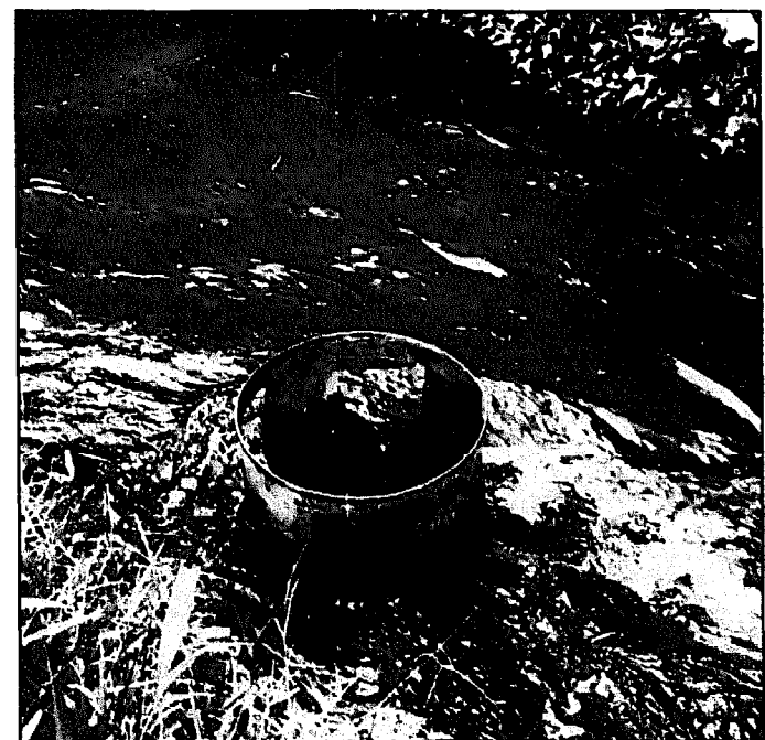
Fig. 5.188. A shaft spillway improvised from an oil drum.
