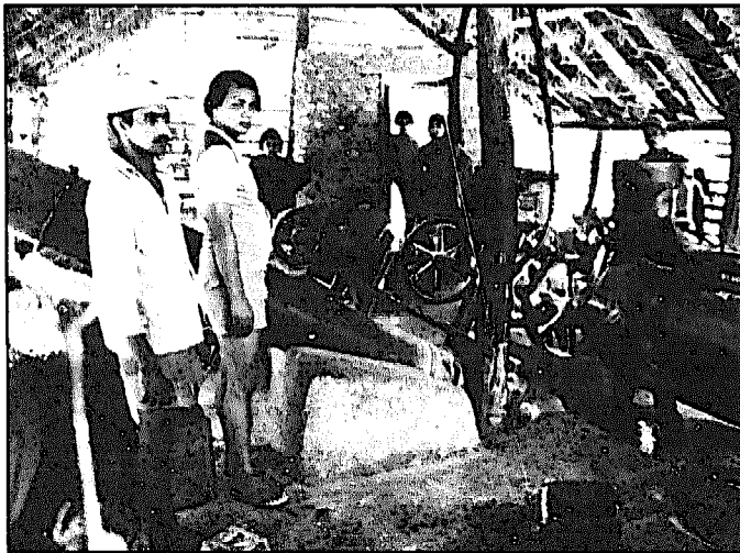
Fig. 10.16. At Ampchaur, the turbine is placed below floor level.
