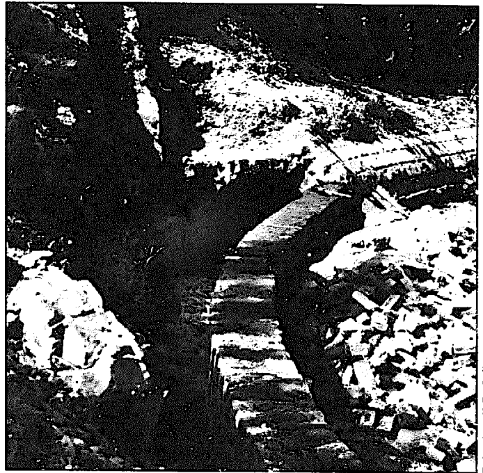
Fig. 5.108. An irrigation canal is covered with a brick arch to prevent slides from obstructing the flow of water.
