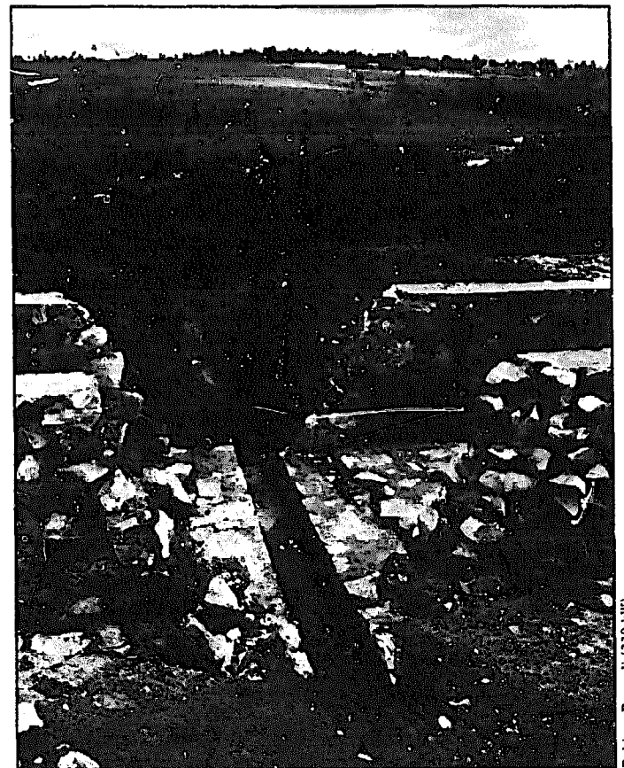
Fig. 5.84. A drainage ditch will eventually pass under the bottom of the power canal. At this site, the portions of the canal incorporating the drainage ditches are completed last.
