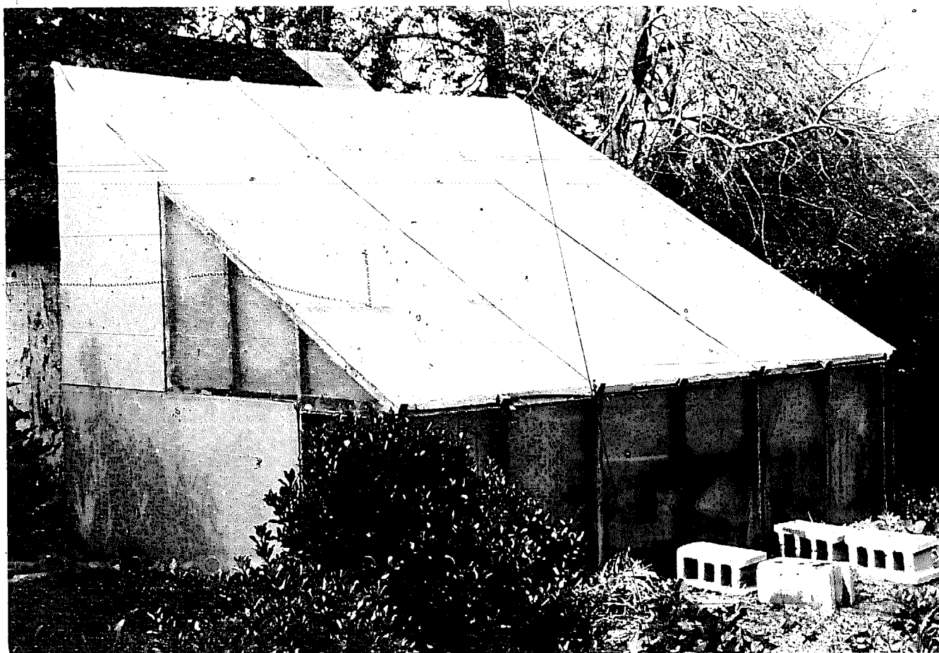
Photo 8-30: Freestanding greenhouse. Long Island, New York.
