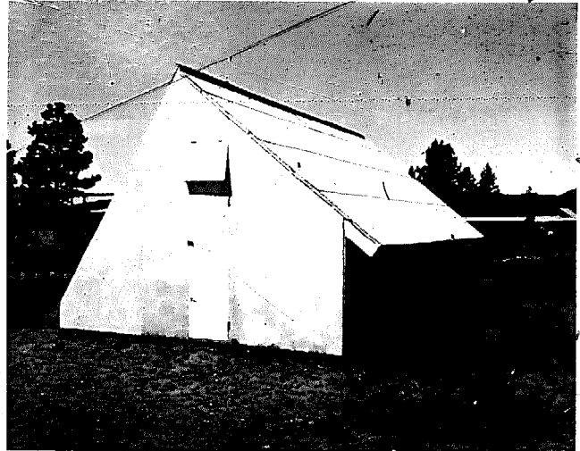
Photo 8-4: Rear roof detail.
