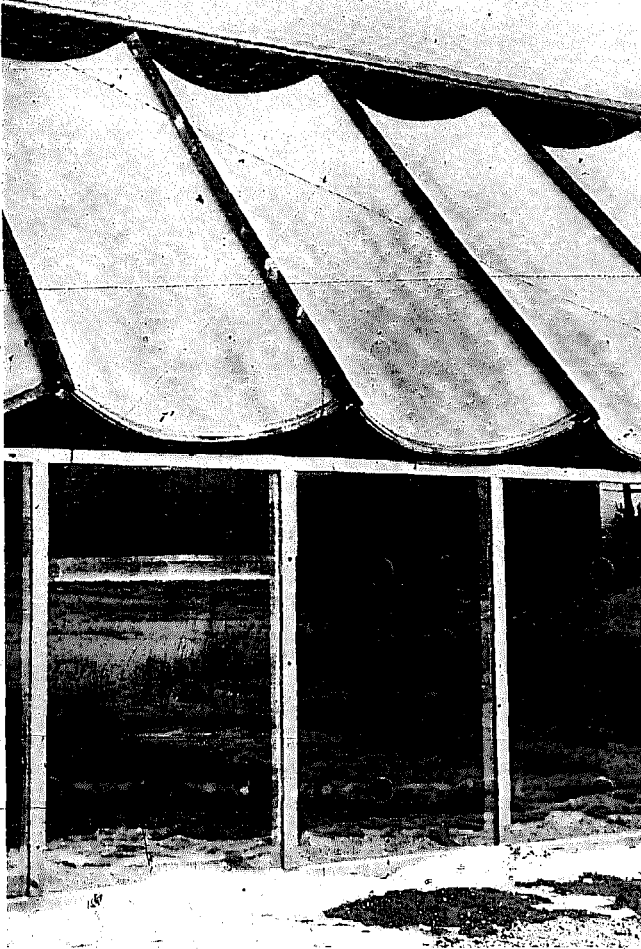
Photo 4-1: Alternate fiberglass glazing method, installed (New Alchemy Institute).
