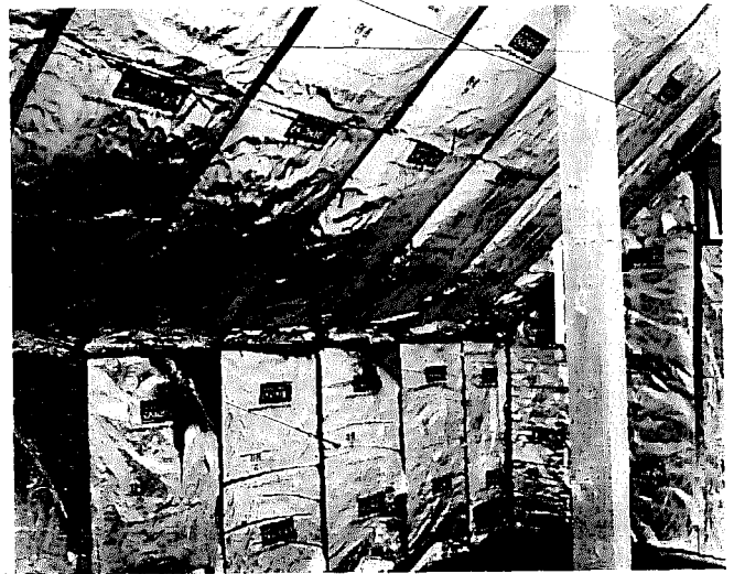
Photo 8-6: Insulation installed. Interior.
