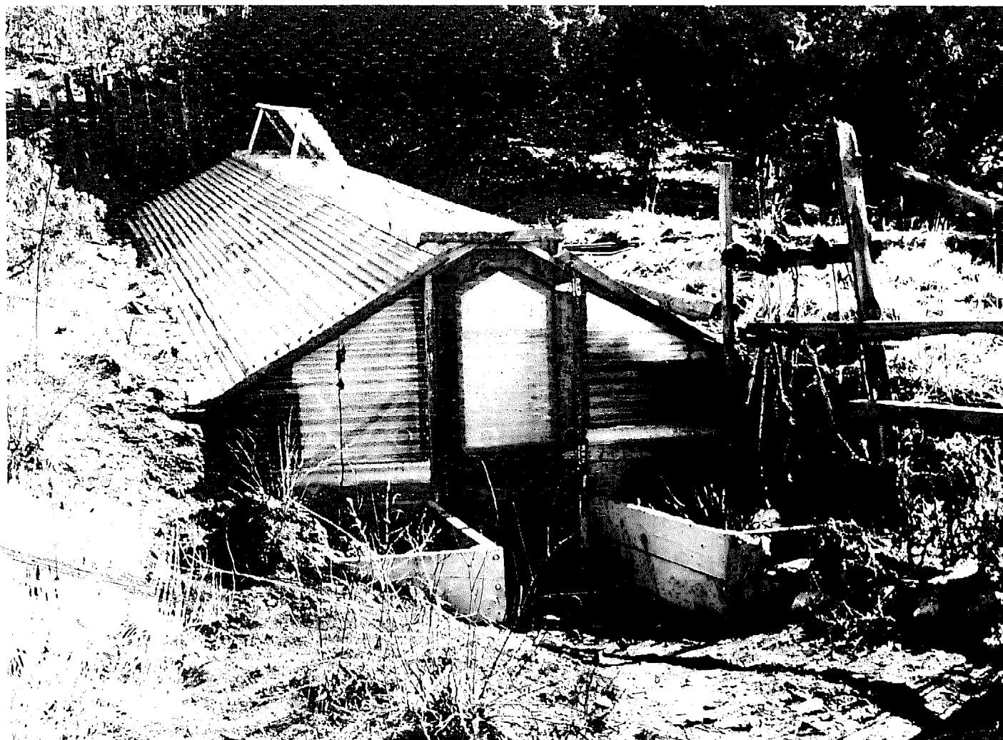
Photo 10-3: The Grouhole as it looks today.
