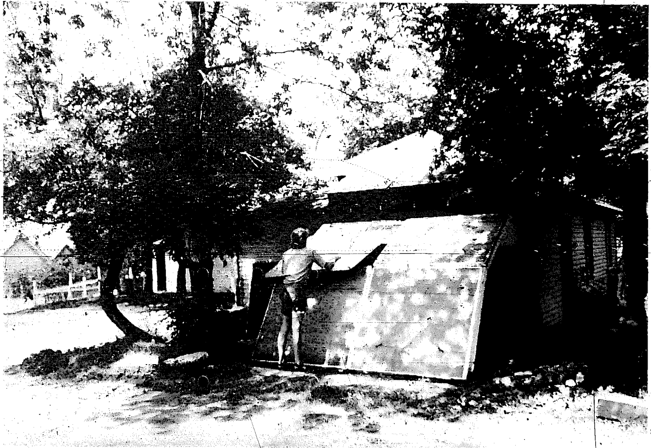
Photo 3-2: Styrofoam insulating panels: attached pit. Milwaukee, Wisconsin.
