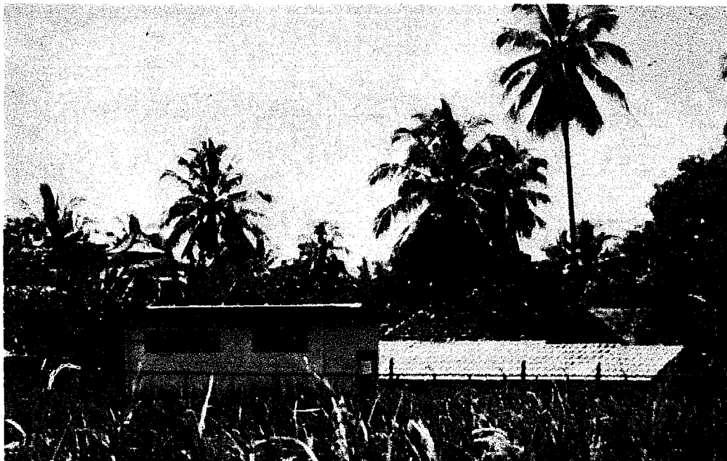
Figure 6.3 5.5 kWp PV Array at Picon, Indonesia
