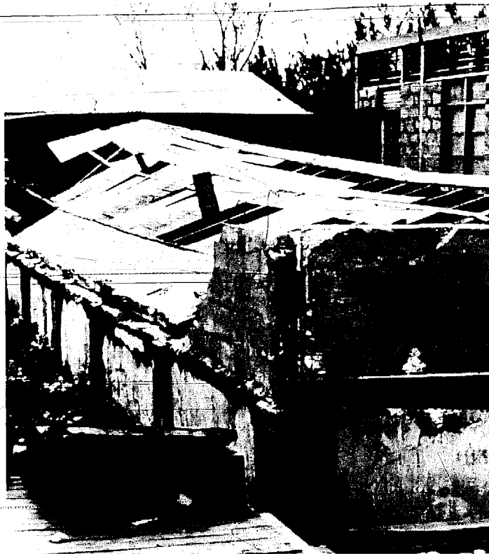
FIGURE 8 COLLAPSE OF ONE-STORY BUILDING CAUSED BY THE NOVEMBER 1974, TYPHOON IN THE PHILIPPINES.
