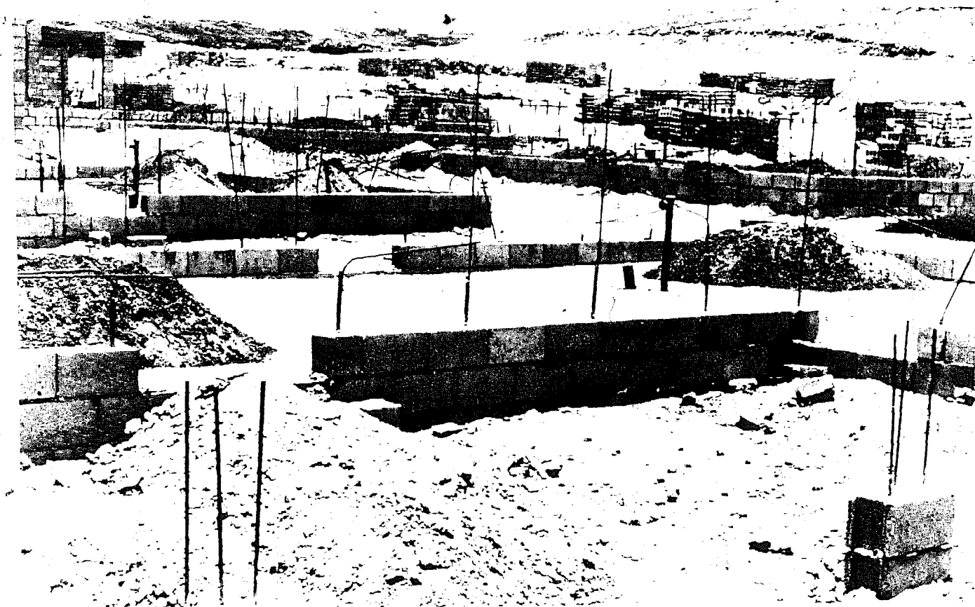
FIGURE 24 REINFORCED CONCRETE MASONRY WALLS UNDER CONSTRUCTION FOR HOUSING IN CENTRAL LUZON, THE PHILIPPINES.
