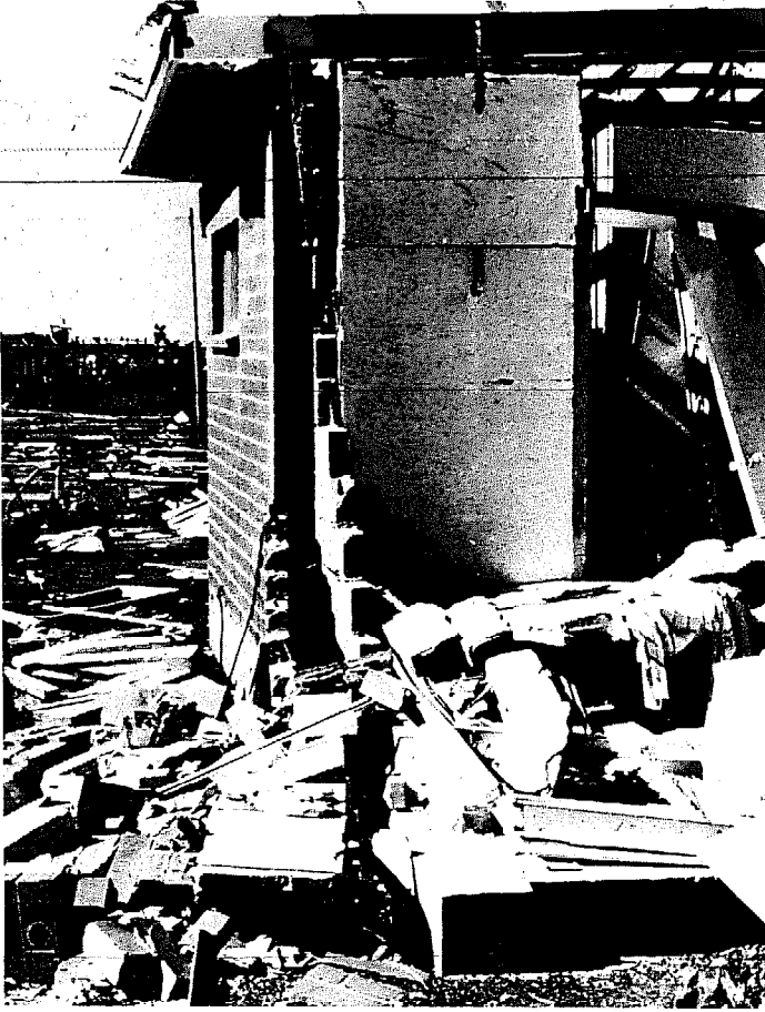
FIGURE 15 BUILDING OF CAVITY WALL CONSTRUCTION IN DARWIN, AUSTRALIA, PARTIALLY DESTROYED BY THE DECEMBER 1974 CYCLONE.
