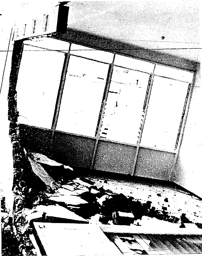
FIGURE 13 INTERIOR DAMAGE OF SINGLE FAMILY HOUSE CAUSED BY THE NOVEMBER 1970 TYPHOON IN THE PHILIPPINES.
