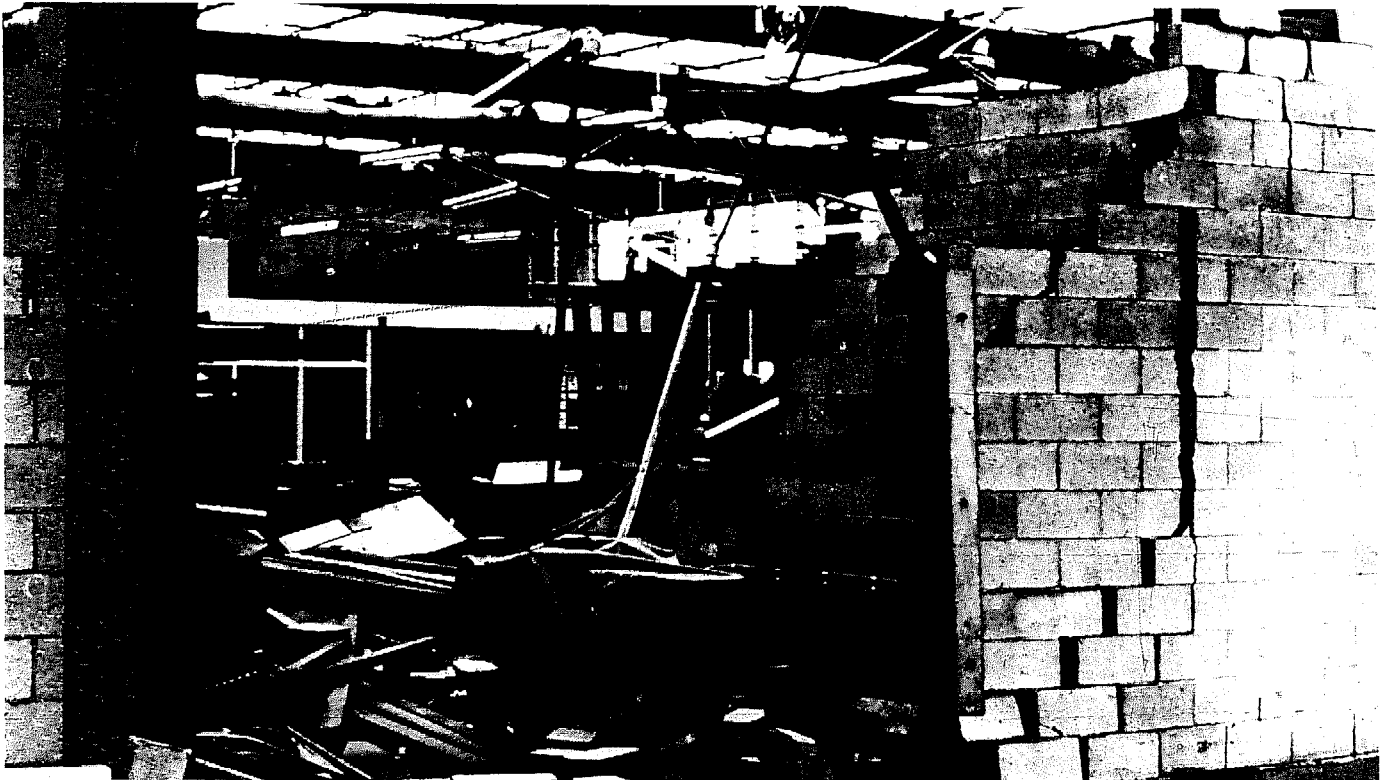
FIGURE 16 BUILDING IN DARWIN, AUSTRALIA SHOWING PARTIAL COLLAPSE OF ROOF AND MASONRY INFILL WALLS CAUSED BY THE DECEMBER 1974 CYCLONE.
