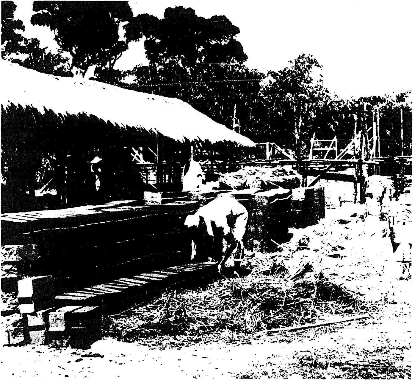
Figure X. 700 Soil-Cement Blocks per Day Were Made in a Hand Operated Machine at Ho Hsiang, Taiwan.
