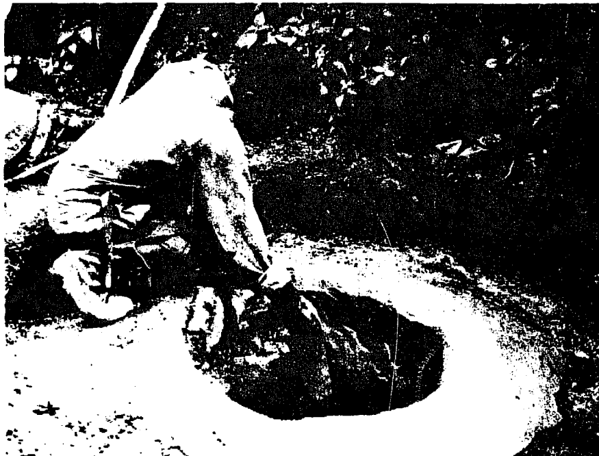
FIGURE C-1 A final layer of mortar is added to an improved storage pit. (Figures C-1-C-3, Robin A. Boxall, Freedom from Hunger Campaign, Ethiopia)
