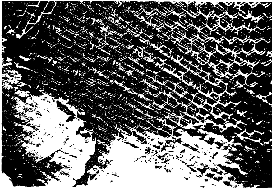
FIGURE 19 Fresh mortar applied to multiple layers of chicken-wire mesh on a 45-foot boat—showing the low-moisture mix that produces a watertight structure. (Noel D. Vietmeyer)
