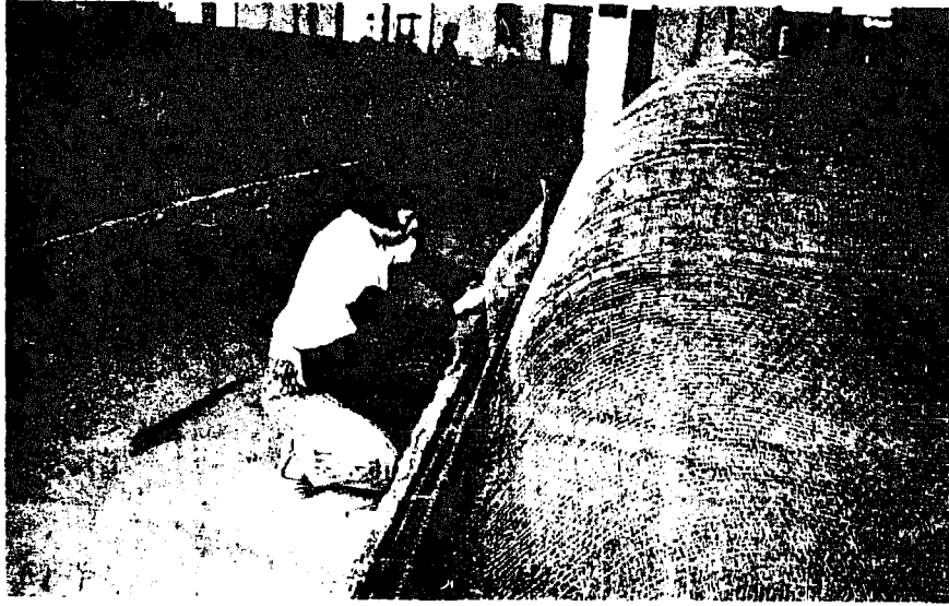
FIGURE A-5 Wire mesh is stitched to the underlying frames.
