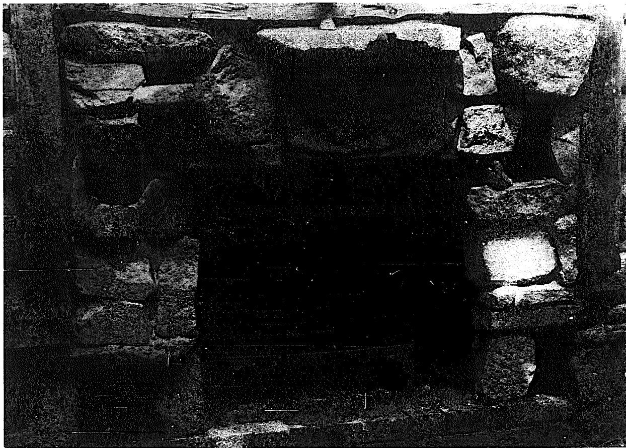
Stone covering a metal firebox.
