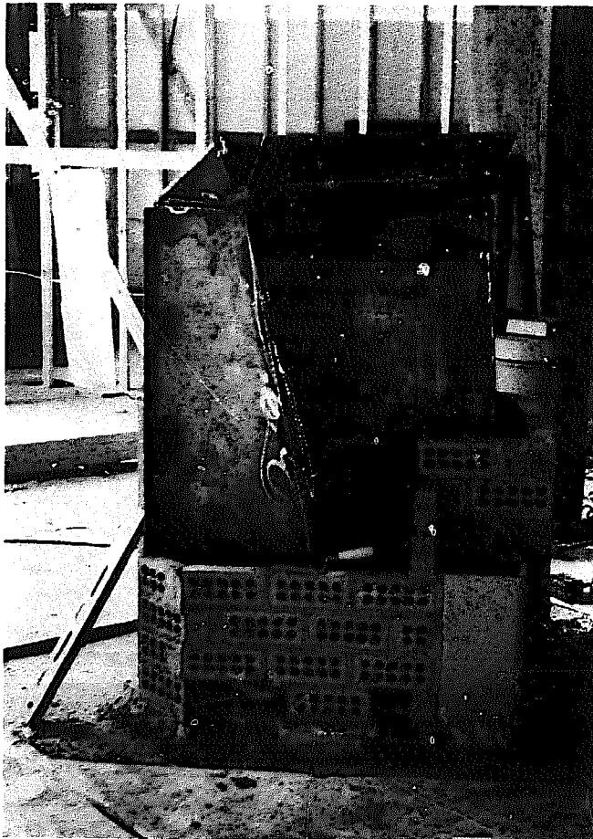
Baffles omitted on this fireplace.
