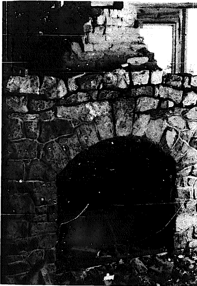
Brick expansion chamber built.
