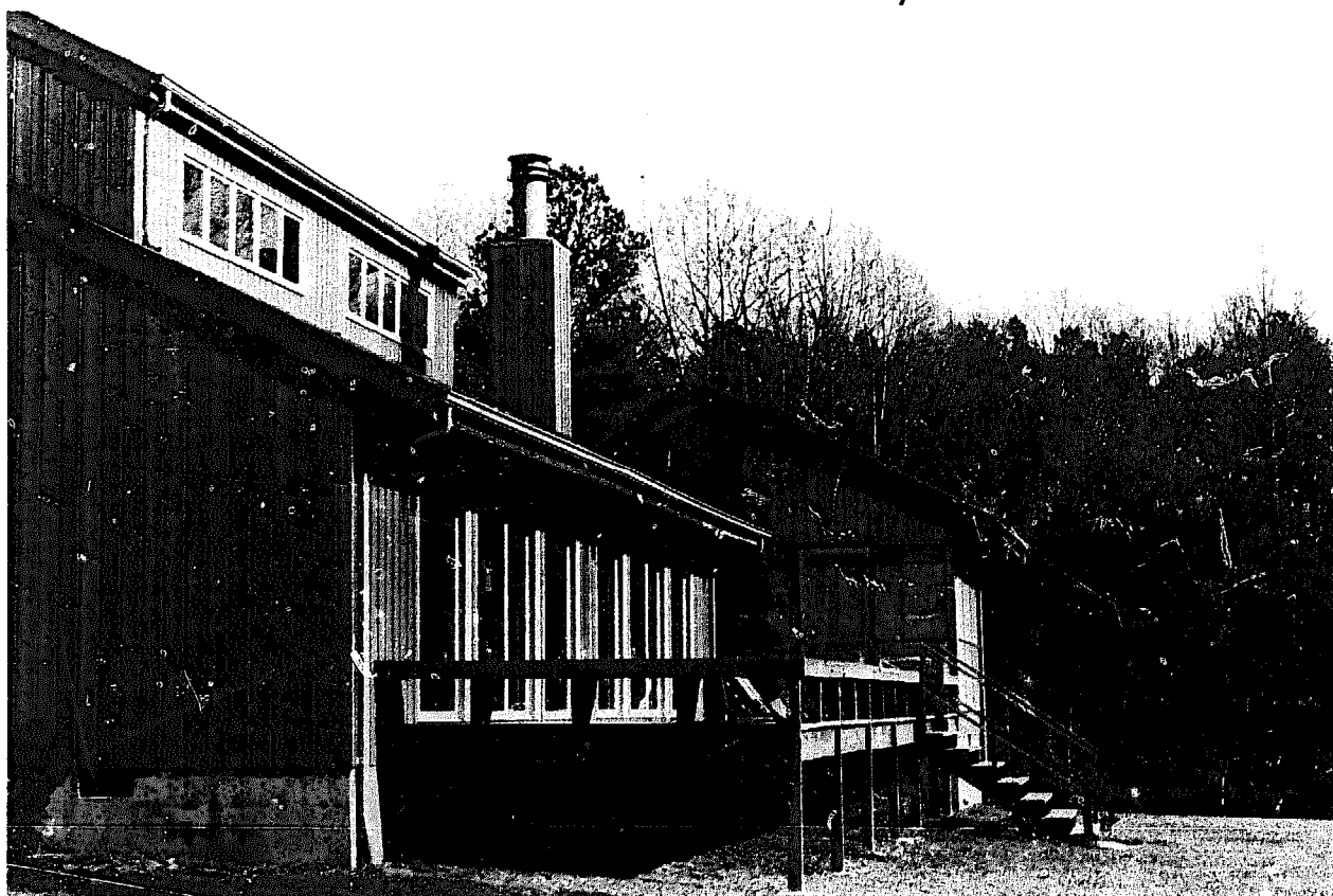
A metal flue in a wood framed chimney.
