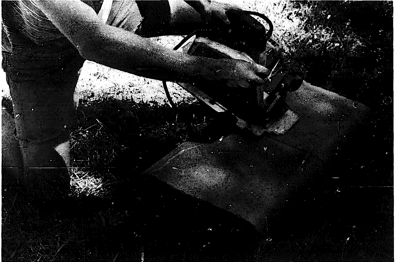
Cutting a flue liner with a masonry saw blade.
