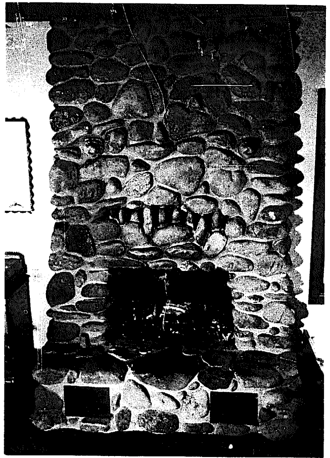
Fireplace built with a commercial heat jacket.
