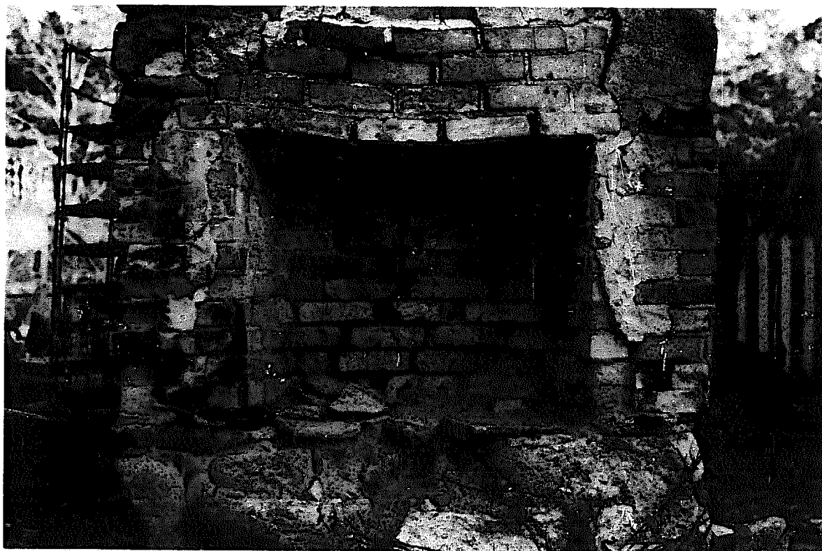
Burned out mortar.
