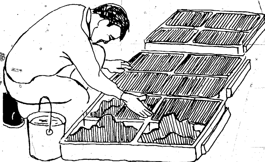
Figure 40. Kneading and leveling the blocks.
