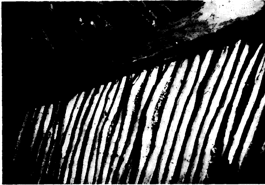
Figure 87. To compensate for the unevenness of the tops of the vigas, saplings can be placed diagonally for sheathing. Note the straw used in this case to prevent the earth fill from sifting through the ceiling.
