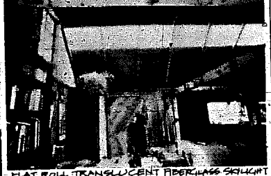
FLAT ROLL TRANSLUCENT FIBERGLASS SKYLIGHT
