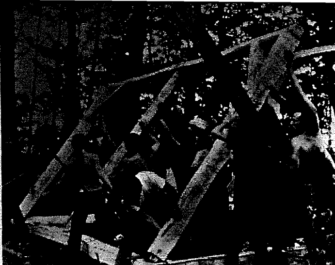
Second frame assembly being raised. Frames in place - 2 safety ropes, each direction. Temporary brace is nailed in place before where assembly is upright in place, braces are nailed to hold it.
