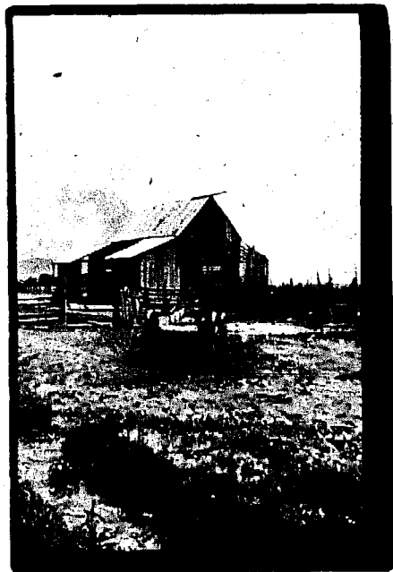
Log barn, Utah
