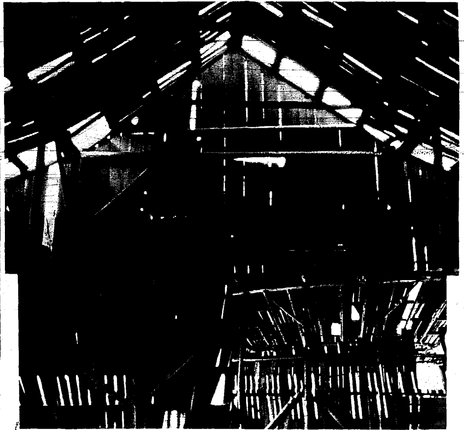
100 year old Barn near Santa Rosa, Calif. Redwood saplings were nailed together. Flate poles were added off on top and bottom, but posts and braces were left round.
