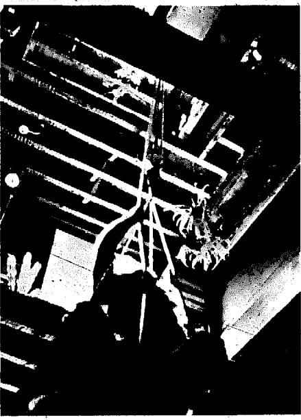
CENTRAL SHAFT CUT THRU 4 FLOORS AND SKYLIGHT INSTALLED IN ROOF. HAND POWERED OAK CHAIR ELEVATOR.
