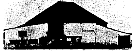
Polygonal barn in Quebec, an extended octagon with lean to's added on.
