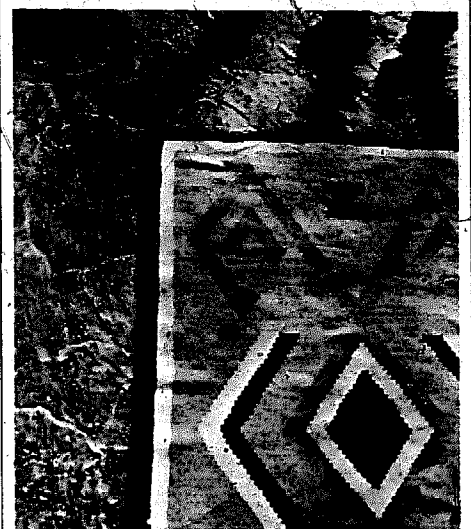
Earth and linseed oiled floor in New Mexico
