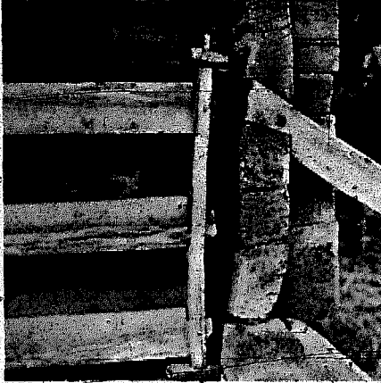
Noisbed wall planks are supports for gate and bannister.
