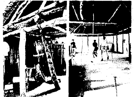
100 year old Barn near Santa Rosa, Calif. Redwood saplings were nailed together. Flate poles were added off on top and bottom, but posts and braces were left round.
