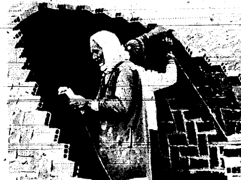
Ghorfa vaulted structures in Tunisia. Originally as grain storage lockers for nomad tribes, now being used for living. Making vaults.
