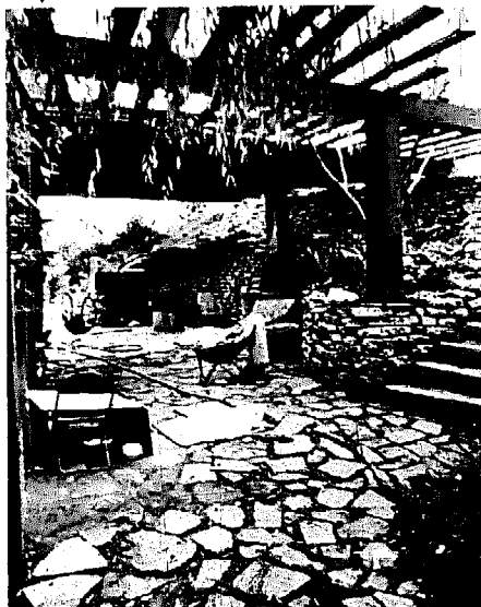
Salvaged chunks of concrete slab used for floor and retaining walls built by Bob Larson.
