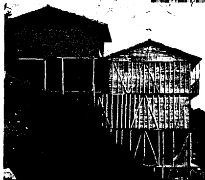
PLASTERED BAMBOO FRAME HOUSE, COLOMBIA. INTERIOR, RUDR HUT.
