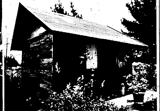
A 8'x13' Gabled building built with all used materials.
