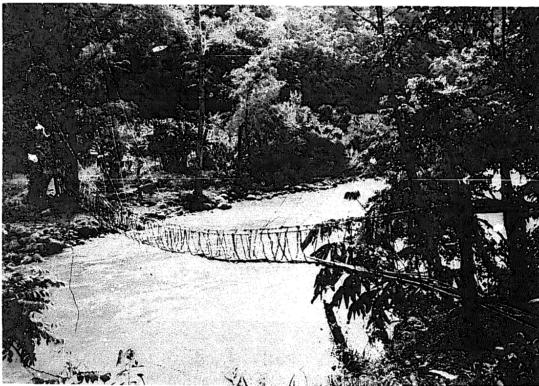
Fig. 53 Kapolame Bridge (from the south bank of the Kaugel River).
