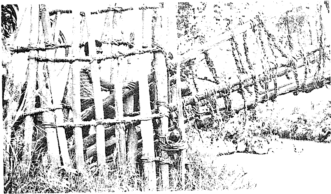
Fig. 74 The south abutment, looking west, Kopeme Bridge.
