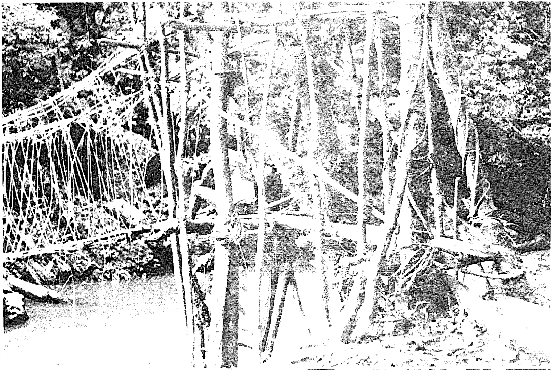
Fig. 123 Anchorage and approach, Iamdelmin Bridge.
