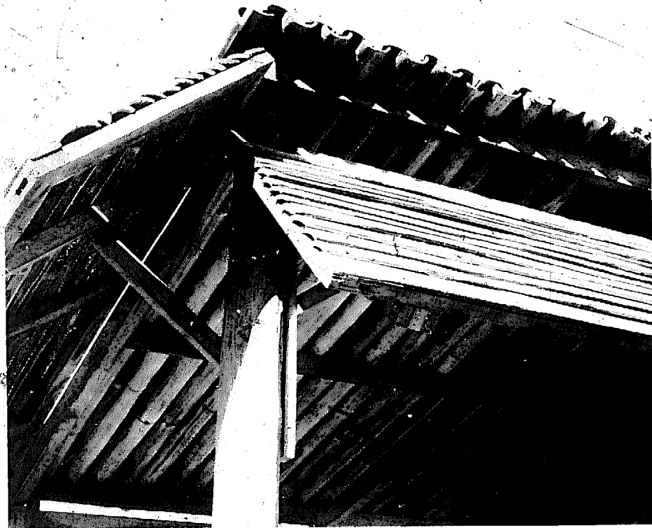
Figure XXIII. Bamboo tile roof of a hut at the Forest Research Institute, Dehra Dun, India
