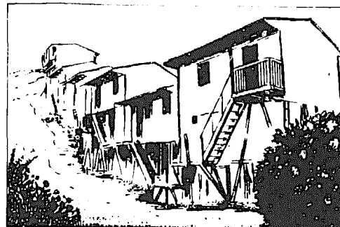
Guadua houses under construction in Manizales, Colombia, by CRAMSA, a local corporation dedicated to appropriate technology.
