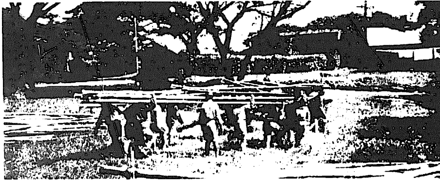
Carrying the Truss to the Site
