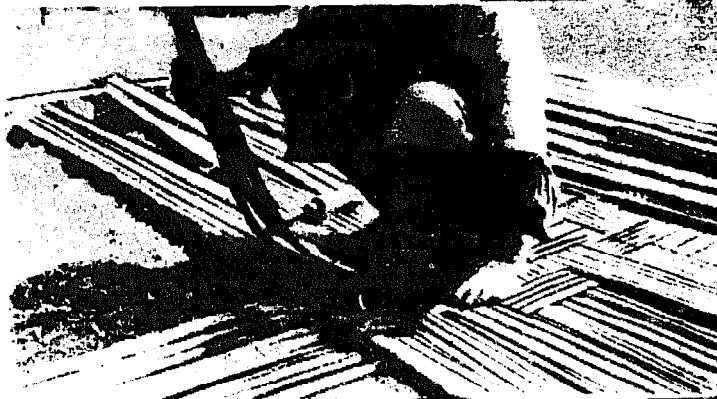
3. Fabricating walling from split bamboo.
