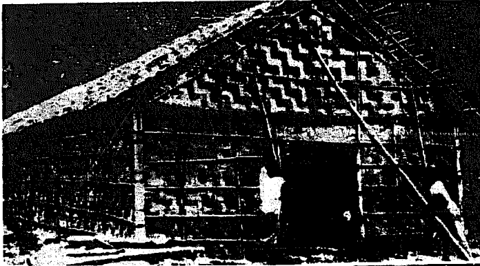
7. Placing end gable.
