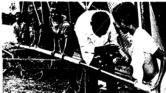
2. The drilling operation
