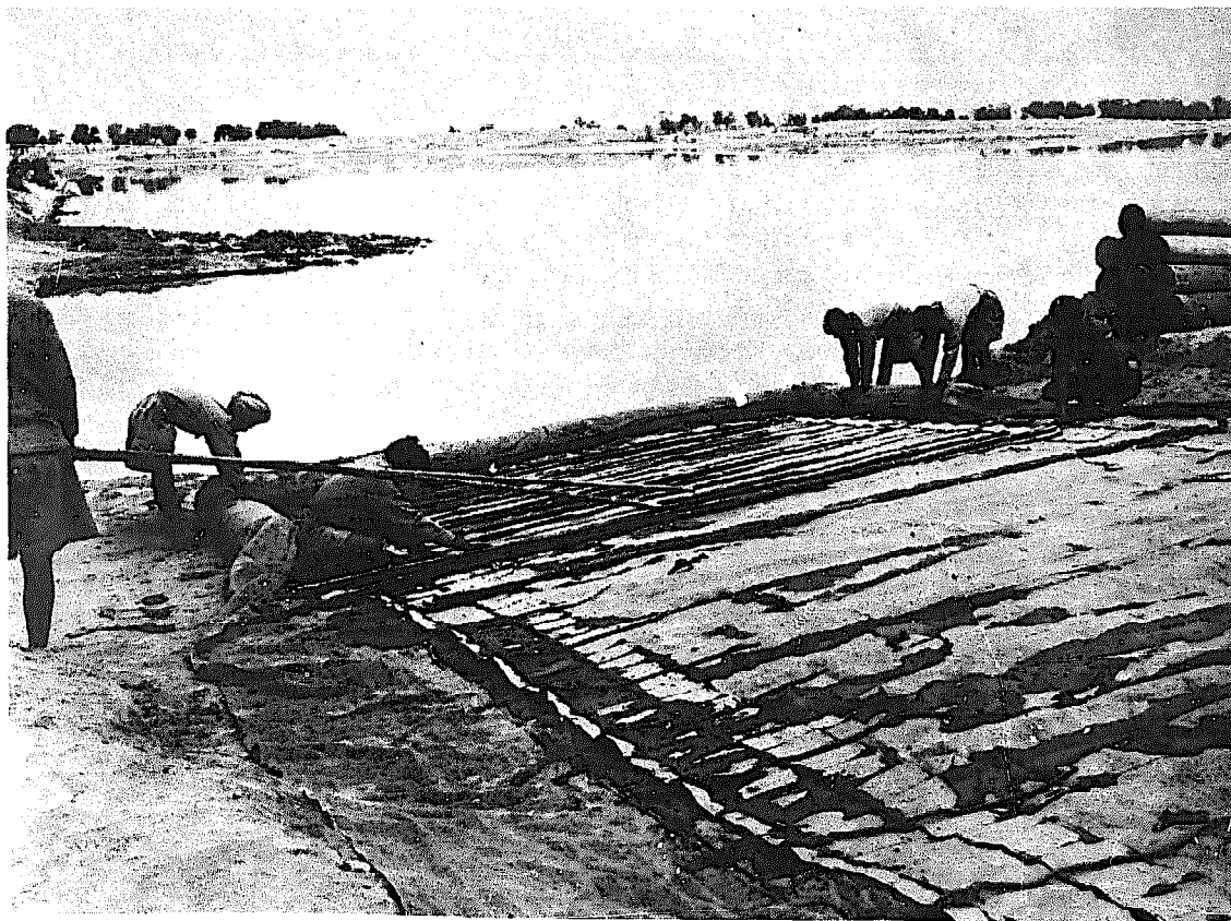
Photo 1. Bamboo inserted into the matbridge.
