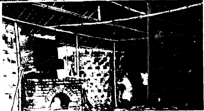
8. View of interior of partially completed building.
