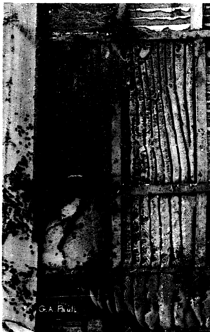
Bees will sometimes occupy the space between the siding and the inner plaster walls of a building, as here shown. The combs at the right are store combs. Bees occupy the space next to the entrance at the left. —
