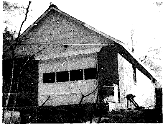
The Garman honey house, a size for the 500-700 colony operator. A five foot loading dock and the overhead door is shown.
