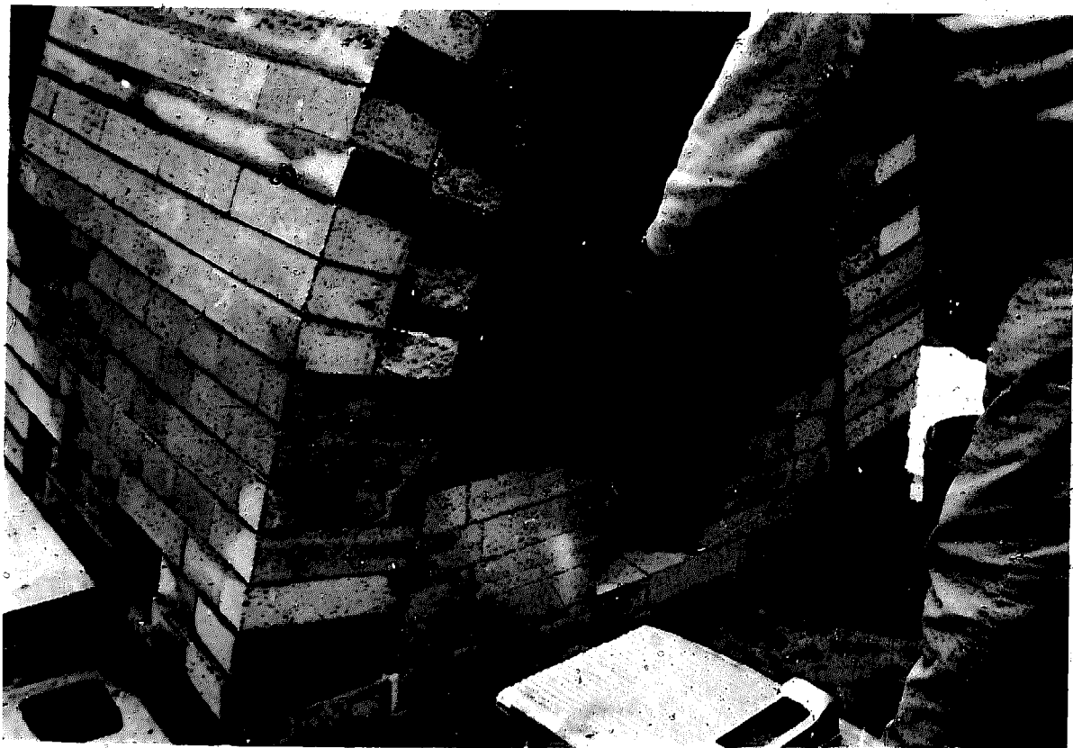
189-A. Building the back wall.
