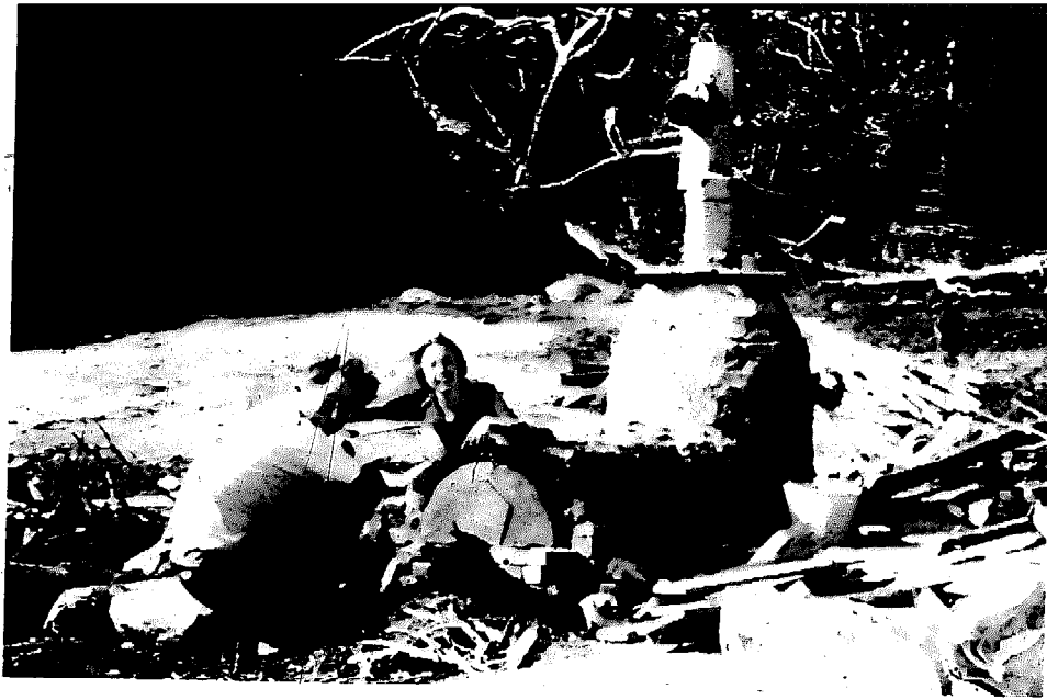
62. Temporary wood burning kiln built by students at the Haystack School, Deer Isle, Maine. Photo by Michael Cohen.
