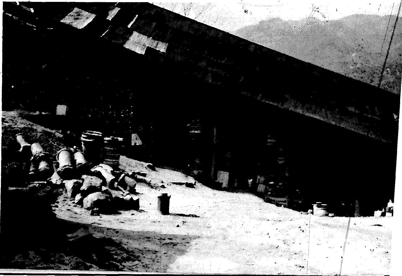
23. Kiln in Shigaraki, Japan. The Shigaraki kilns have an unusually steep slope.
