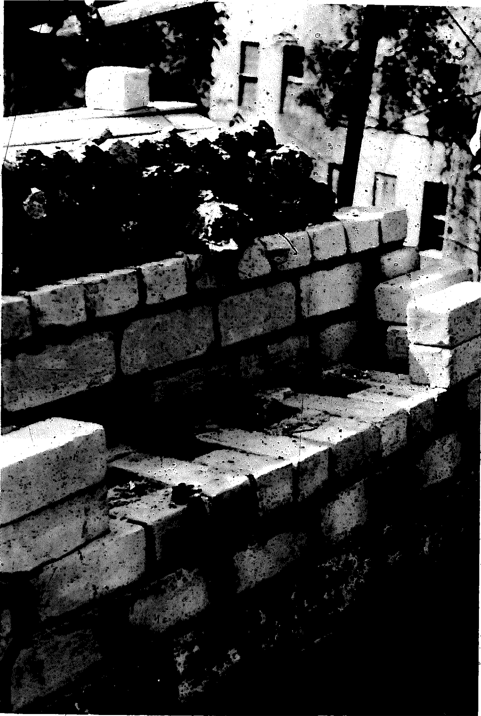
202. Back wall of the third chamber, with flues. The construction of the arch from cylindrical brick can be seen.
