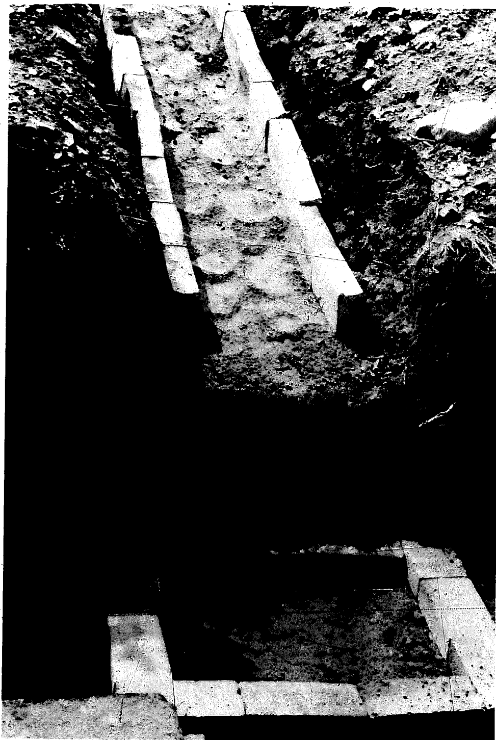
177. Starting the walls of the trench and the firebox. The bricks are placed directly on the ground.
