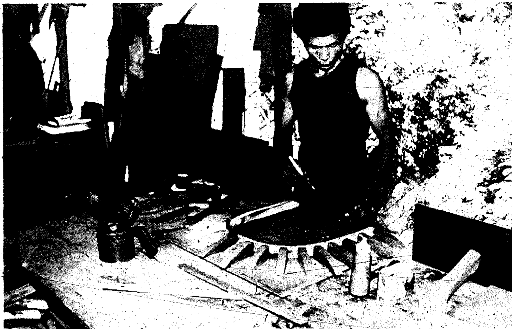
Figure 32. Moulding U-shaped components (Note kerosene fired torch used to assist with severe bends)
