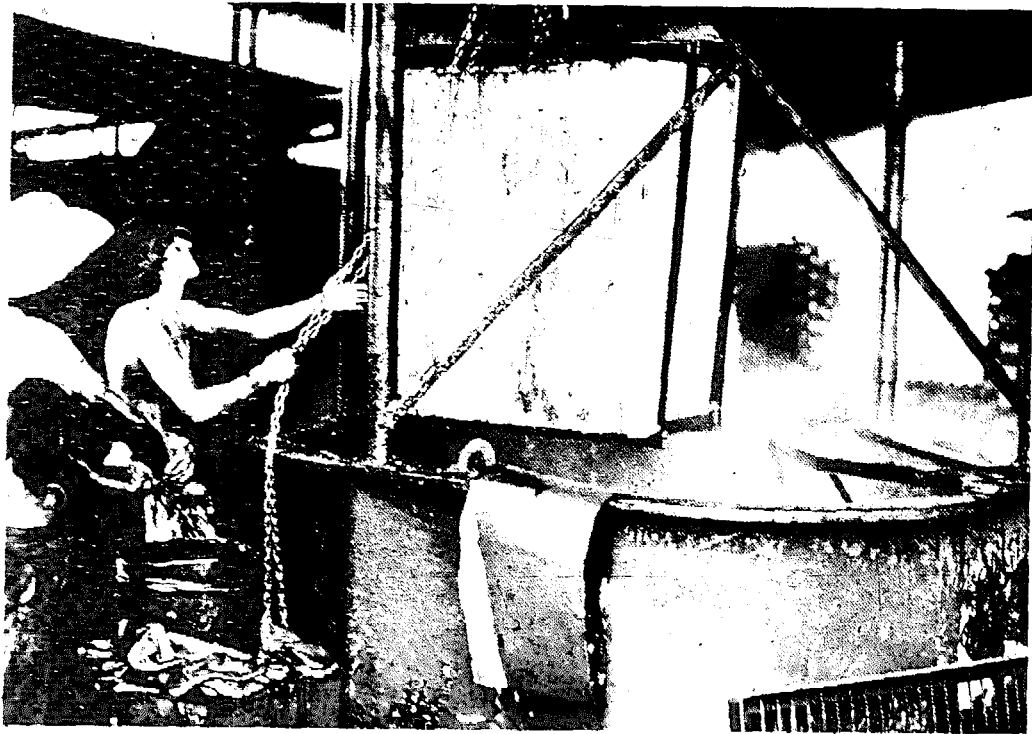
Fig. 12a Manufacture of asphalted roofing sheets.. Dipping in asphalt. Note the use of a steel cradle and chain-operated hoist. The operators wear gloves to protect their hands but their bodies are covered in asphalt due to working stripped to the waist in the heat. A wise employer would insist on light cotton shirts and provide a laundry service.
