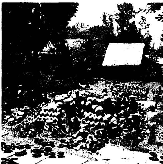
Fig. 2-7: Top layer of the Sinde kiln is laid.
