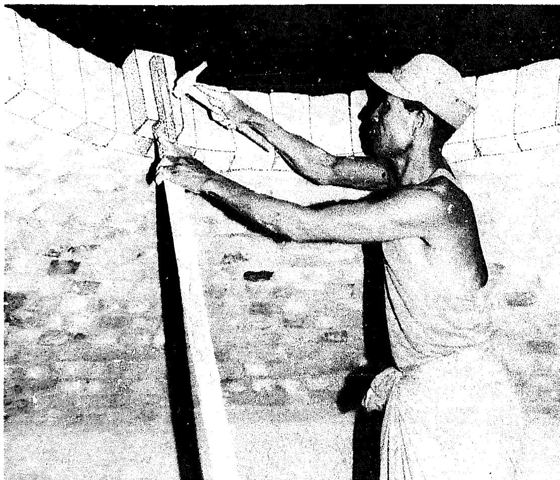
Fig. 2-98: Construction of a dome
