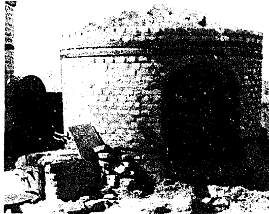
Fig. 2-21: First chamber of Bujora kiln. Water and oil pipes lead to the three fireboxes.
