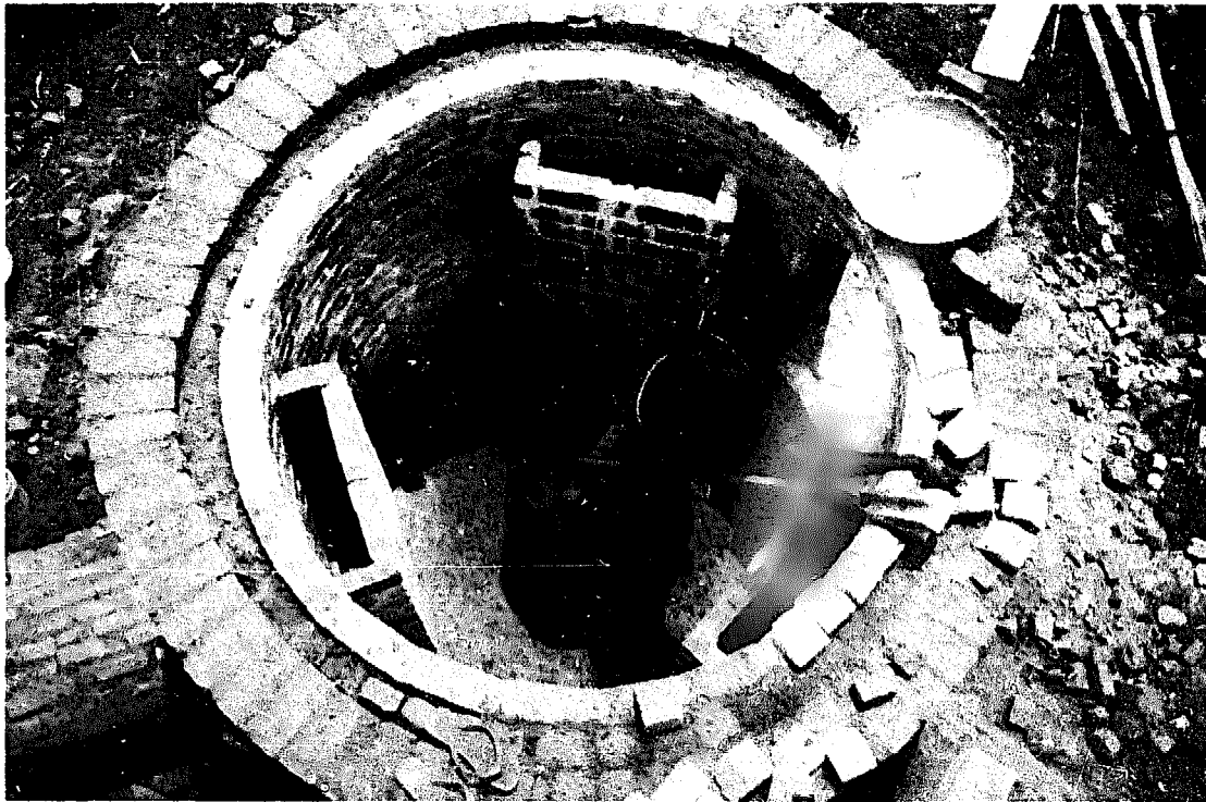
Fig. 2-101: Starting the dome of the Bujora kiln. Note the insulating loose layer between the inner firebrick lining and the outer wall. The bagwalls proved to be too high and were later cut in half.
