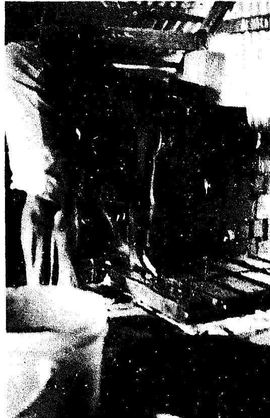
Fig. 1-35: Slop-moulding of bricks
