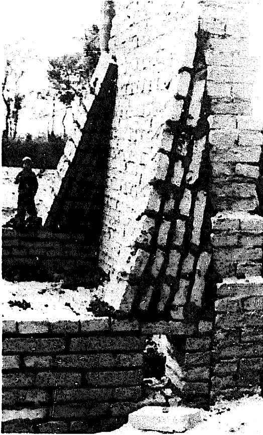
Fig. 2-105: Construction of a catenary arch without support. Beginning of construction. Nepal.
