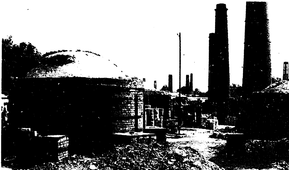
Fig. 2-18: Circular coal-fired down-draught kiln. Khurja, India.
