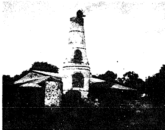
Fig. 2-22: The Bujora kiln seen from the other side with its chimney chamber to the right
