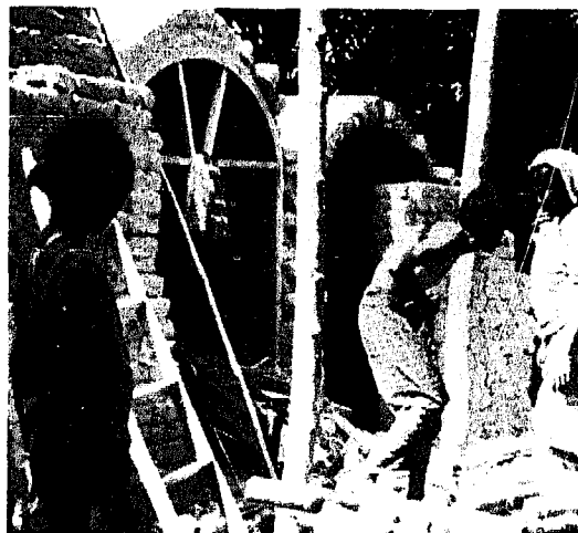
Fig. 2-32: Two-chambered kiln built with sun-dried bricks. Suvapur, Bangladesh.
