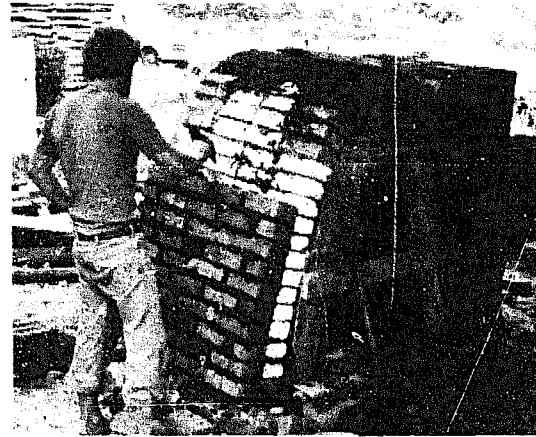
Fig. 2-104: Catenary arch under construction. Singisi, Tanzania.
