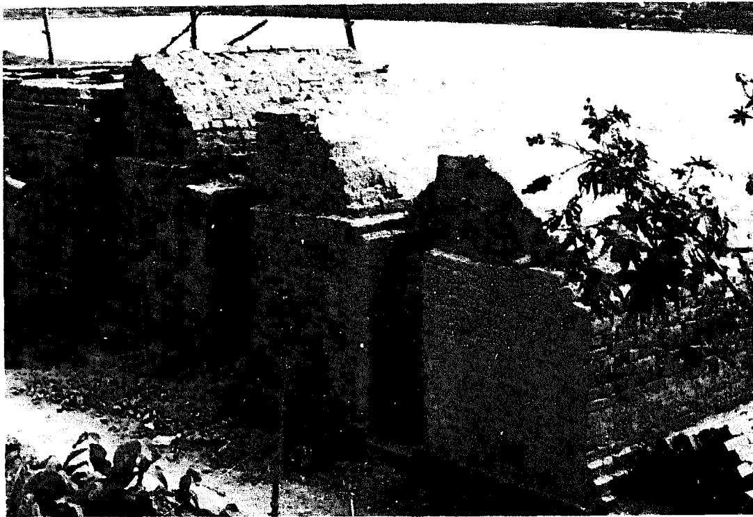
Fig. 2-31: Three-chambered wood-fired kiln under construction. The firebox to the right and the chimney at the other end are not yet ready. Champaknagar, Bangladesh.
