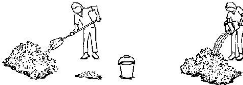
Mix the fine soil with the filler and the water
